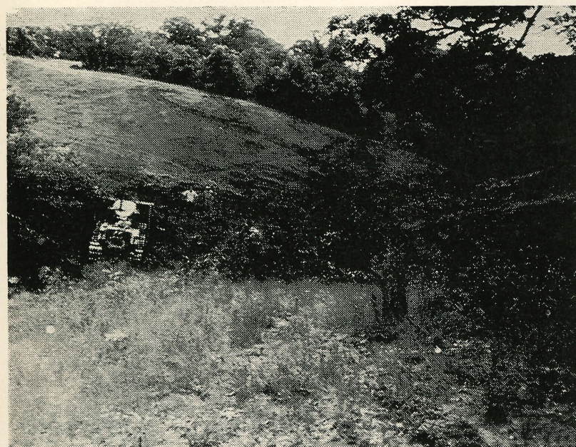
Carl Proctor, Contractor of Blakesburg, Iowa, clearing site for a drop-inlet structure on George Leffler farm.
