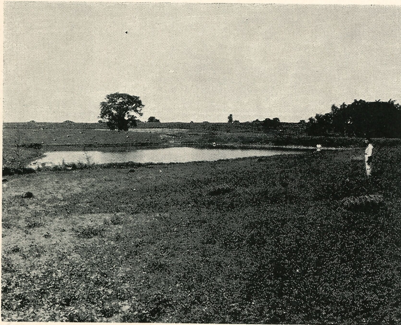
Pat Corbin, Soil District Commissioner, viewing Drop-inlet on the Falvey Bros. farm in Wayne Township. This erosion control structure was built to control two severe over-falls. It contains 4600 cubic yards and was completed in 1958. This farm is managed by Mrs. L. A. Falvey, Monroe county's State Representative and operated by Ed Murphy.
