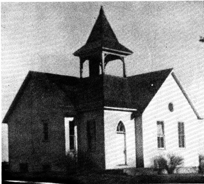
The Liberty Church Building 1907-1941
