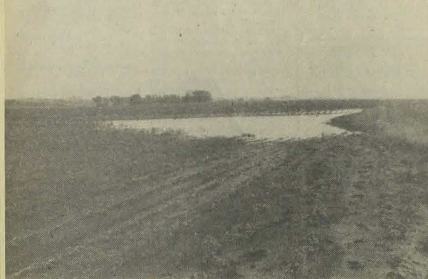
TERRACES REDUCE EROSION: Damage to crops in the recent deluge which afflicted crops in Clarke County was reduced where farmers had installed conservation practices such as the tile intake terrace (above and below). Those without
