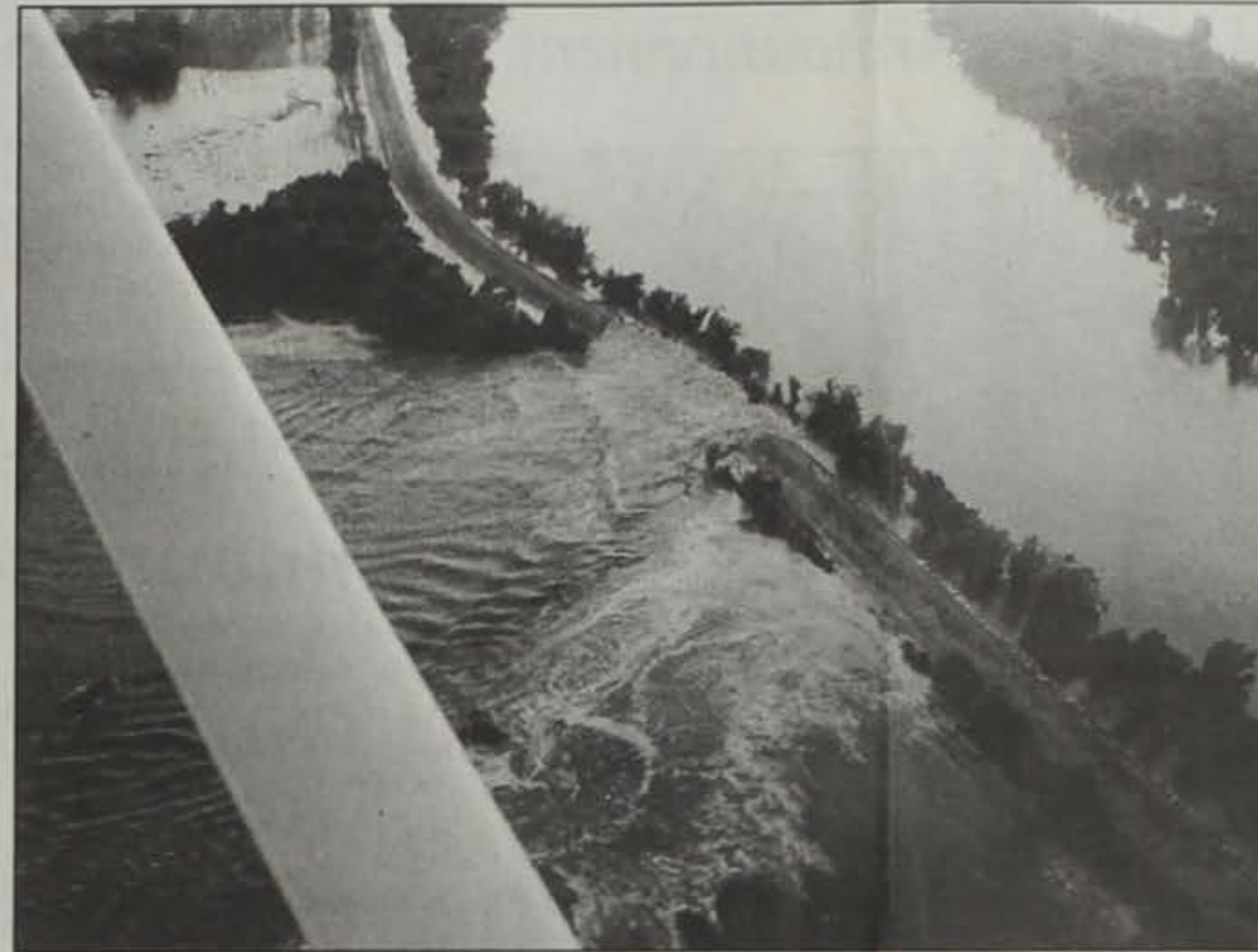
This aerial photo shows the break in the levee southwest of the city of Oakville. The break led to several feet of water in the town, and to the flooding of thousands of acres of farmland (submitted photo).
