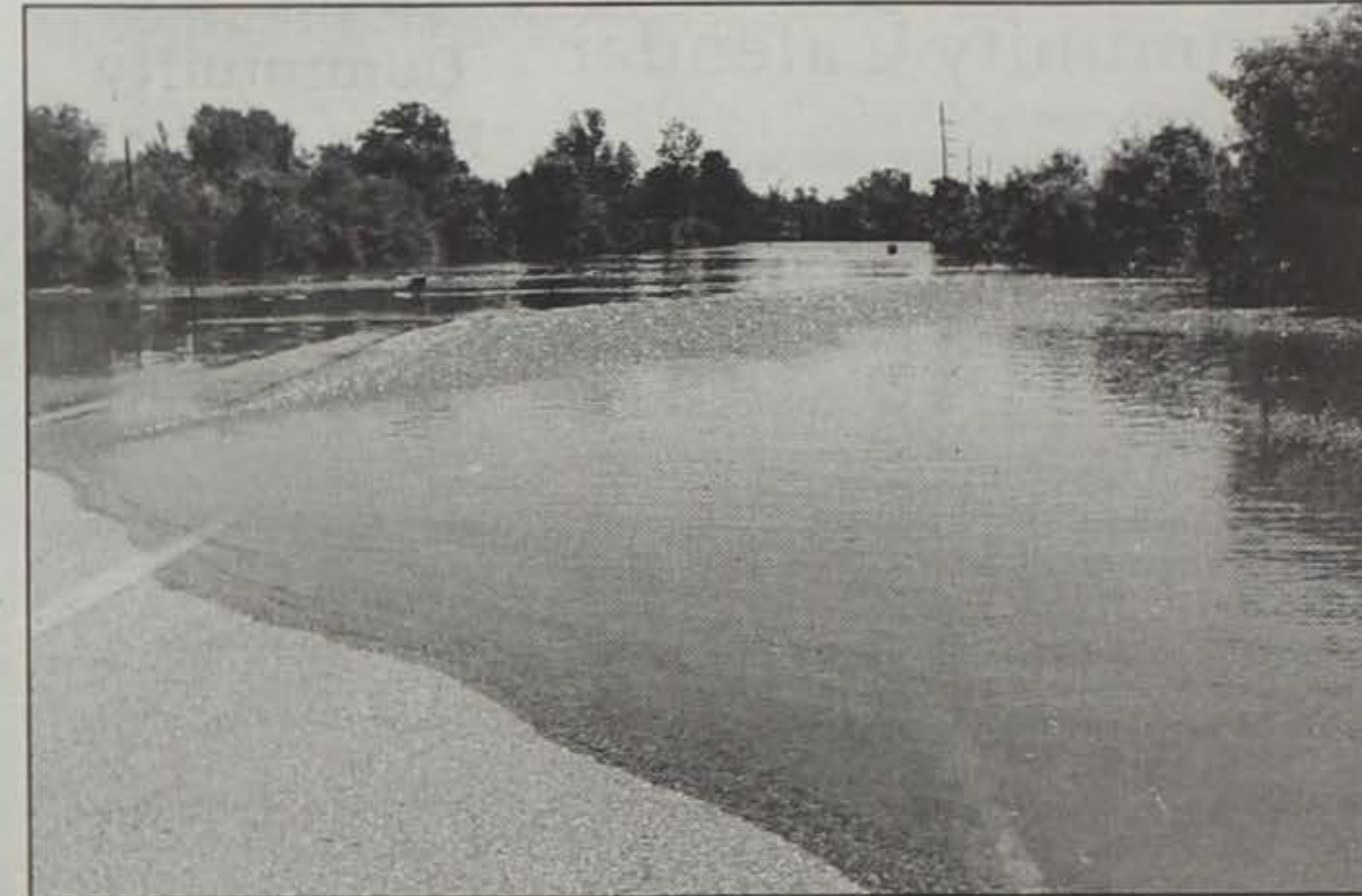
Water gushes across Highway 99 east of Wapello after a levee was compromised last Friday. As of Tuesday afternoon, the bridge east of Wapello and the highway remain closed, although water levels had begun to recede.
