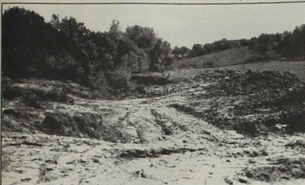
An early view of the gully site on the Dimon project during the clearing of trees and ditch debris.
