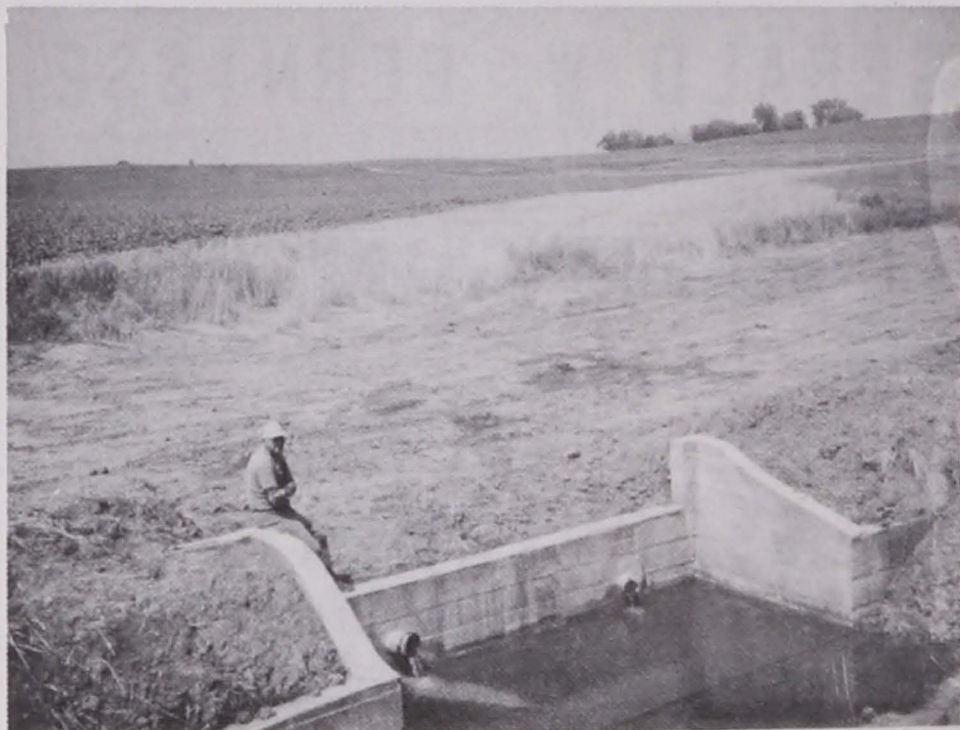
Concrete Erosion Control structure on Gilbert Sonksen farm in Crystal twp.
