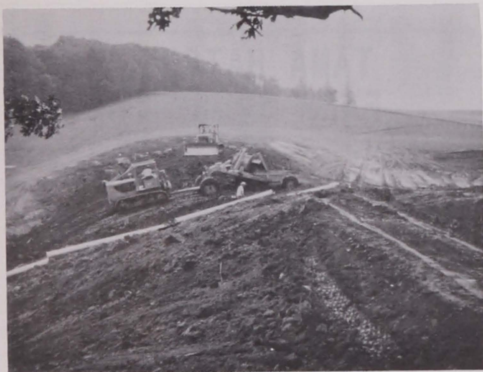
Earth erosion control structure being erected on Laverne Eckhart farm in Spring Creek twp.
