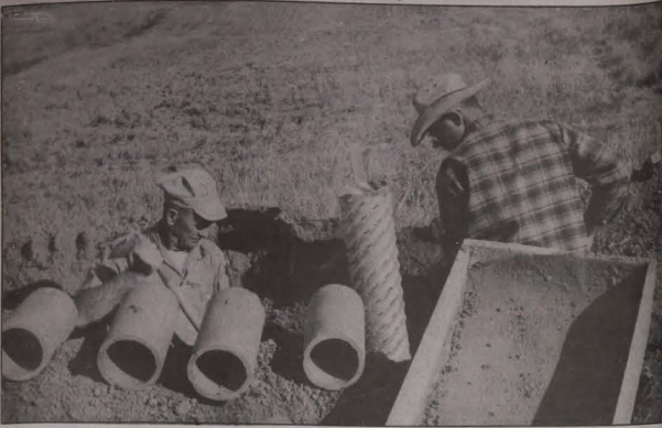
Recognize these conservation farmers? Cleve Bennett (left) and his son Bill Bennett on a farm near Elgin using cement to stabilize a tile intake for terraces.
