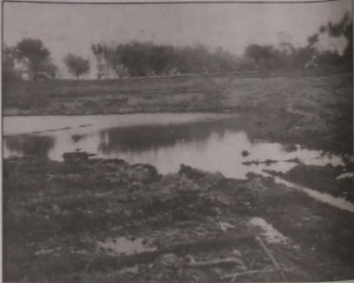
Pond site of Jon Grimes farm located in Union township, southeast of West Union. Site can be seen from Hwy. 56. A 3.5 acre pool area was constructed in the fall of 1995. It's not yet full.
