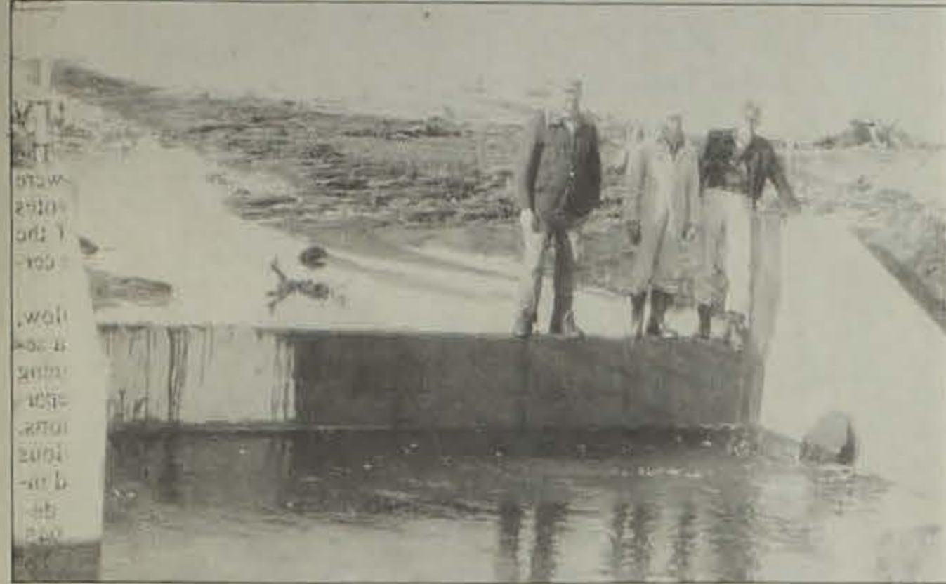
ABOVE: Shown is a reinforced concrete drop structure built in Sept. 1959. The structure helped to stabilize the grassed waterway and provide an outlet for the tile drainage system. Pictured in 1959 are, left to right, the landowners Tony Broghammer and Gib Hoffman, along with the late George Carlson, district conservationist for the SCS at that time. Below: Thirty-five years later, Broghammer and Hoffman are standing next to the erosion control structure still functioning as it was originally designed. (Photo submitted)
