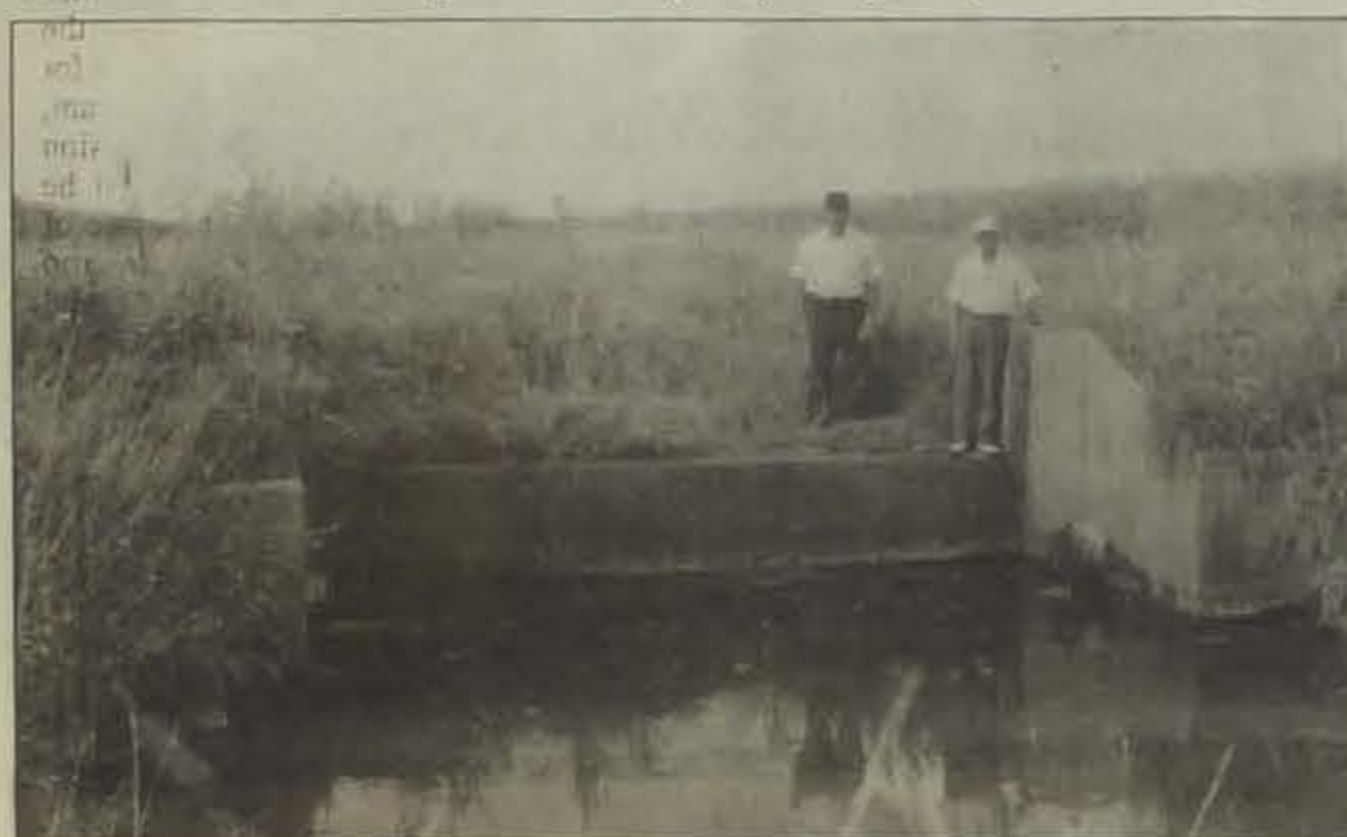
ABOVE: Shown is a reinforced concrete drop structure built in Sept. 1959. The structure helped to stabilize the grassed waterway and provide an outlet for the tile drainage system. Pictured in 1959 are, left to right, the landowners Tony Broghammer and Gib Hoffman, along with the late George Carlson, district conservationist for the SCS at that time. Below: Thirty-five years later, Broghammer and Hoffman are standing next to the erosion control structure still functioning as it was originally designed. (Photo submitted)
