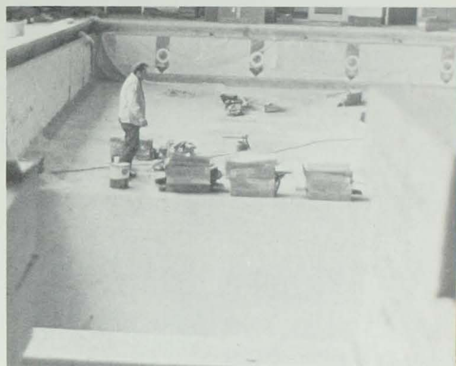
The beginnings of the pool
