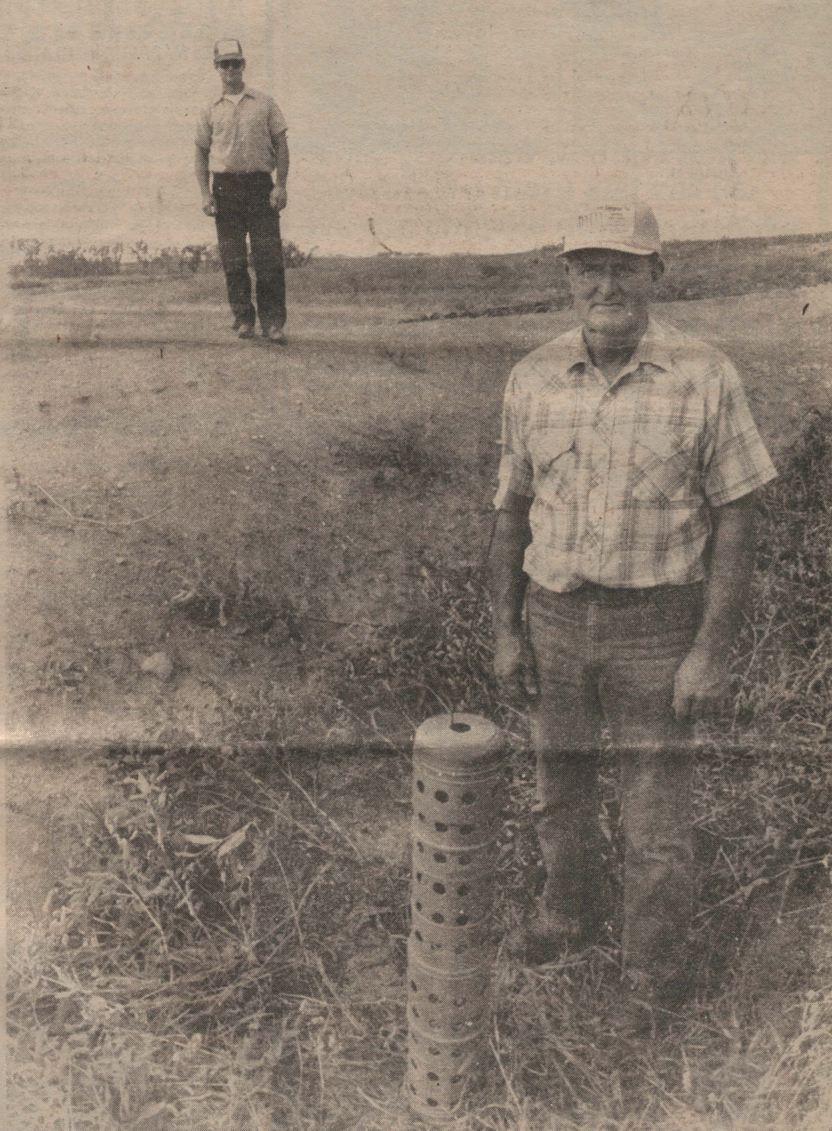
BERNARD KELLEY of Terril stands near the intake to a tile built behind one of several new terraces while his son, Dan, shows the height of the terrace. The Kelley farming operation has constructed approximately a mile of
