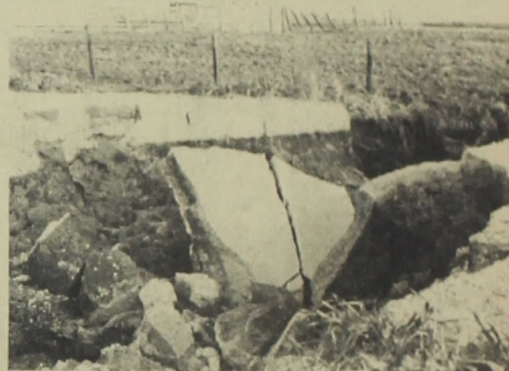
Torrential rains washed out four bridges and over fifty culverts on secondary roads in Louisa county during the weekend. This is a scene about seven miles south of Wapello near the Bernard Gajewski farm.
