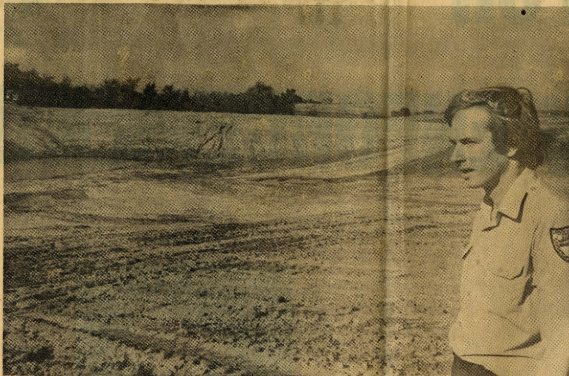
Atherton stands in front of the earth dam constructed to form the four-acre pond that will be
