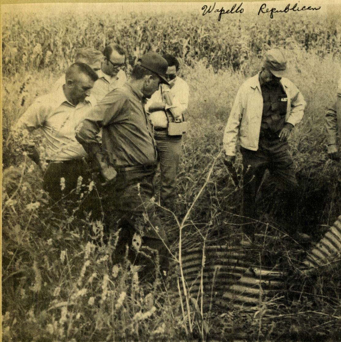
Bill Matthews, (right) soil technician for Louisa County, explains the purpose of a catch basin constructed on the John Hupp farm west of Wapello. Others pictured are Howard
