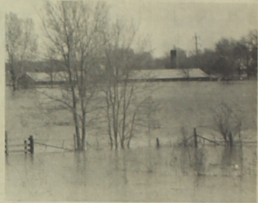
Farm buildings east of Wapello were nearly roof high after floodwaters covered the area. Highway 99 from Wapello to Burlington was closed Monday when water ran across the road.
