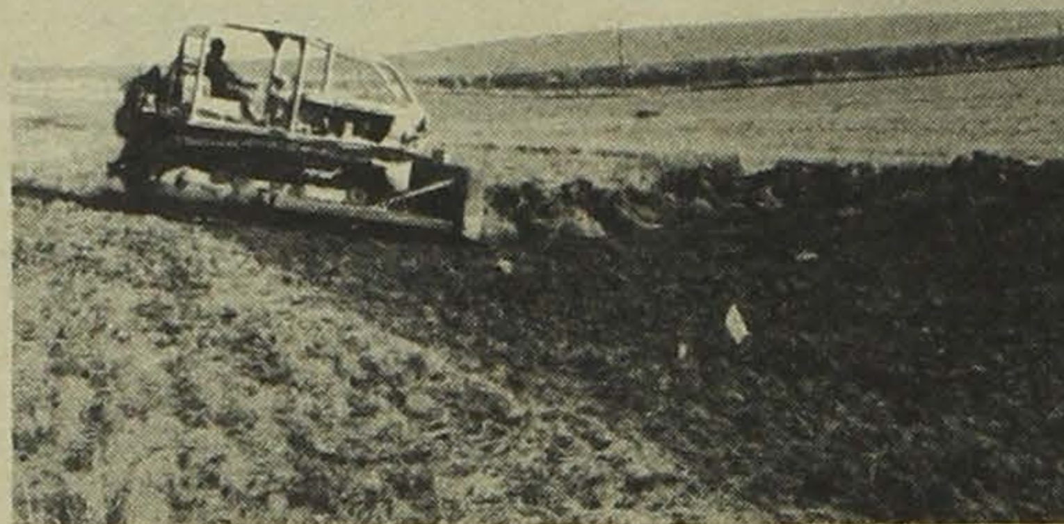
Waterway under construction on the Lawrence Blunk farm in Benton Township.
