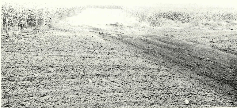
A newly completed watercourse which is an extension of one that a neighbor had built earlier.
