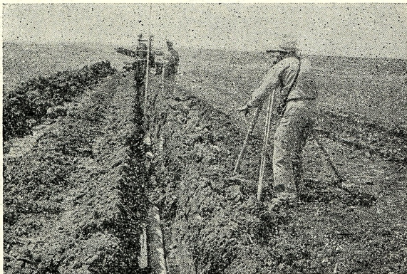
Sac County Soil Conservation District technicians checking tile grade before tile was covered.
