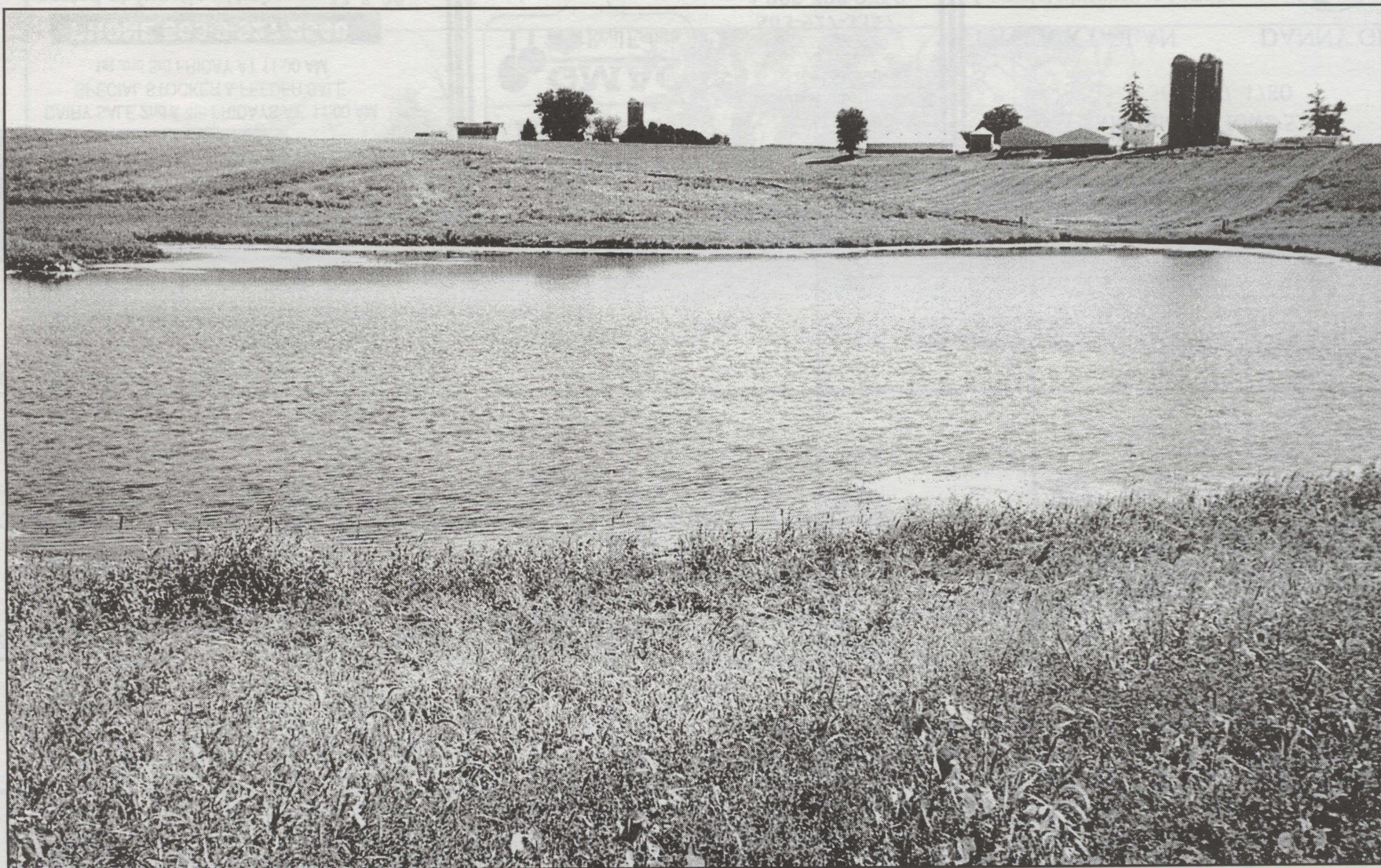
This Grade Stabilization Structure is located on the Walter Westhoff farm in Sec. 34 of Elk Twp. The Elk Creek Water Quality project provides cost share for erosion control and down stream water quality benefits.
