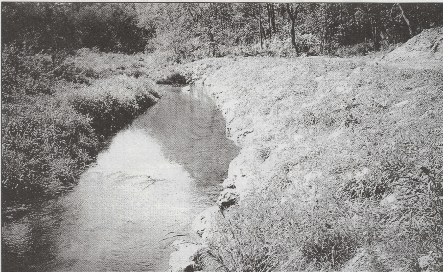
Streambank Stabilization is an important conservation practice to eliminate bank erosion and improve water quality. With assistance from the Wildlife Habitat Incentives Program (WHIP), Mr. & Mrs. Tom Benson were able to improve this stretch of the Little Turkey River. Water quality and trout numbers have improved as a result of this WHIP project.
