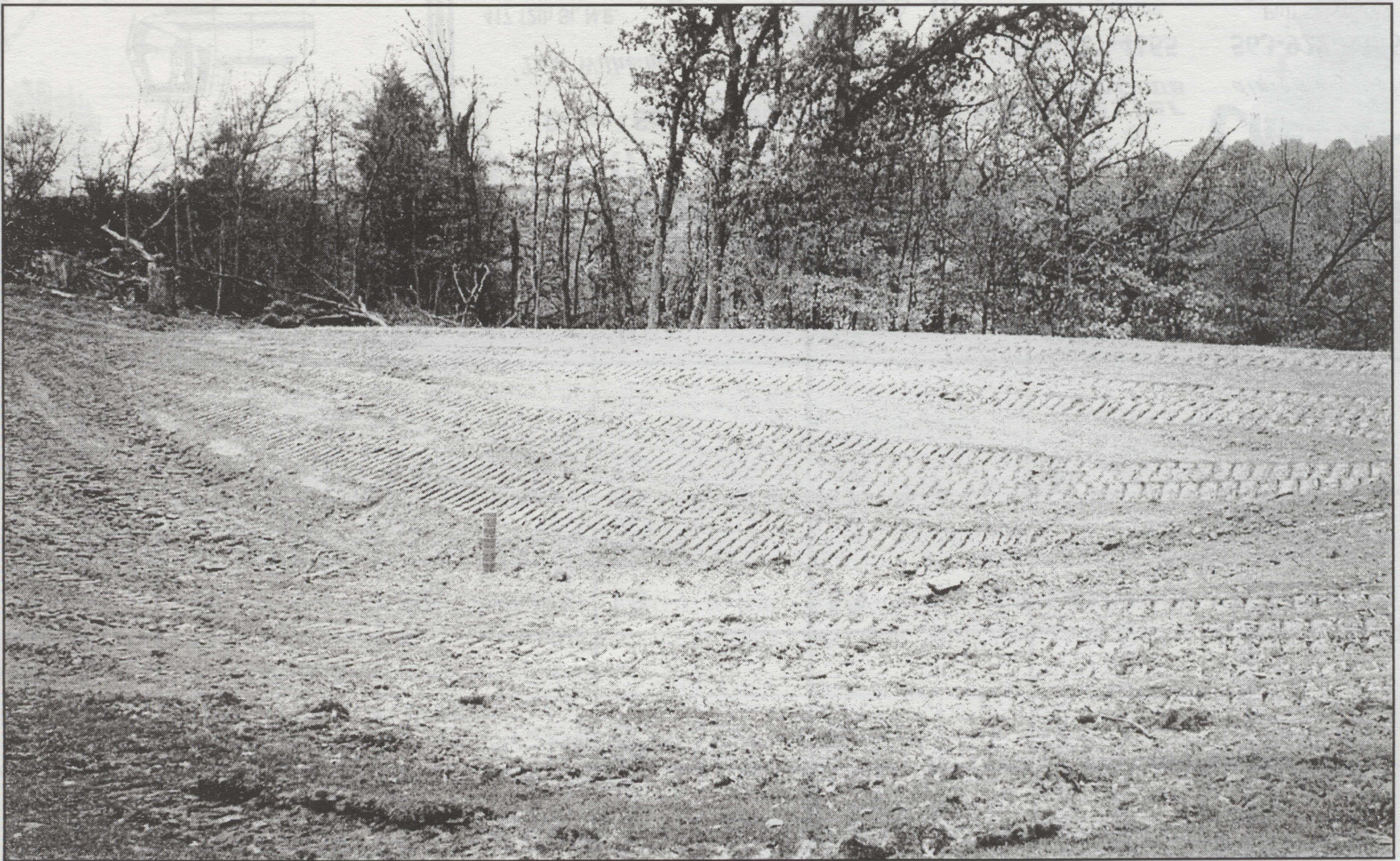
Pictured is a Water and Sediment Control Basin on the Herb and Theresa Sperflage farm in Sec. 1 of Elk Twp. This structure prevents gully erosion. It also traps water and sediment providing protection for the Spring Falls trout stream. Cost Share funding is available through the NRCS EQIP program.
