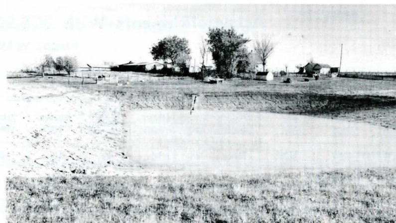
Conservation needs study show that Appanoose County farmers need about 2800 livestock watering ponds such as this one at Clarence Whitehead farm west of Moravia, Iowa. Most ponds also serve to control gully erosion and provide fishing and wildlife areas. Seeding and fencing are needed here to complete this practice.
