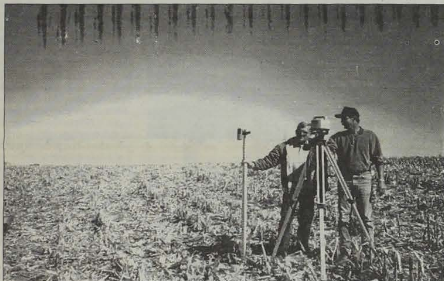
Clair Acker shows Dave Burmeister the ropes in staking out a terrace.
