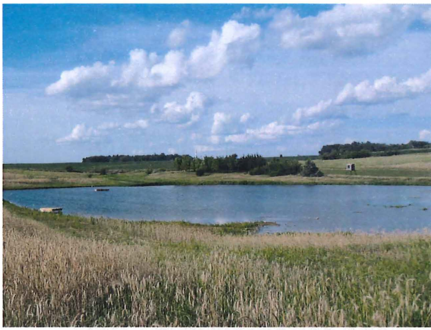
Rick Angell's grade stabilization structure
