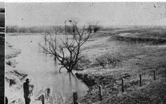
R. Beatty - J. Starceovich farm, Cooper Creek Watershed, east of Centerville. Gully control dam and stock water pond. 4 inch trickle tube pipe here provides 1.6 acres of surface water and 3.5 acre feet of temporary storage. Drainage area is 21 acres. Diversion at right prevents barnlot drainage from entering pond.
