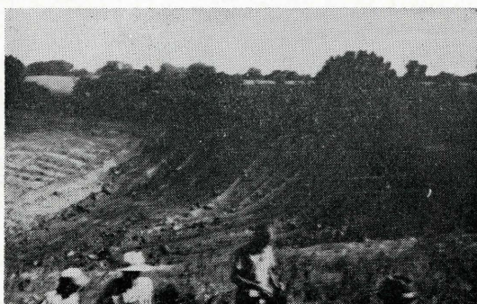
Harold Hawk farm, Iconium Watershed, southeast of Iconium. Farm pond built to furnish livestock water and to also control gully erosion. Regular installation of work such as this is used by the District to also demonstrate conservation practices.
