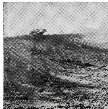
Ward Daniels farm, Moulton Watershed, southwest of Moulton. 12 inch drop-inlet gully control and run-off reduction structure. Run-off rate from 59 acres is reduced 94%. 9 acre feet of temporary storage is provided above the normal pool of 1 acre.
