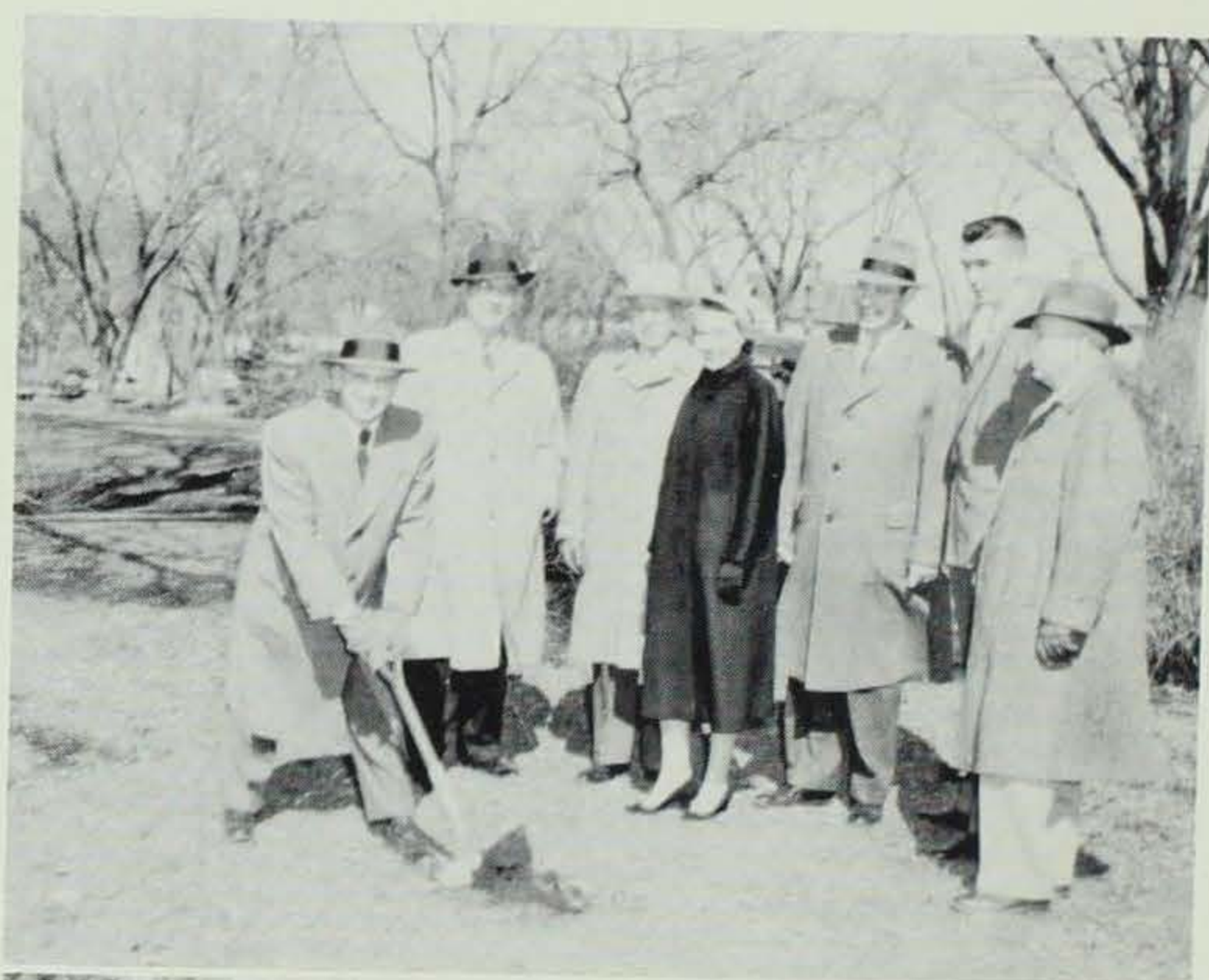
Ground breaking ceremonies...
