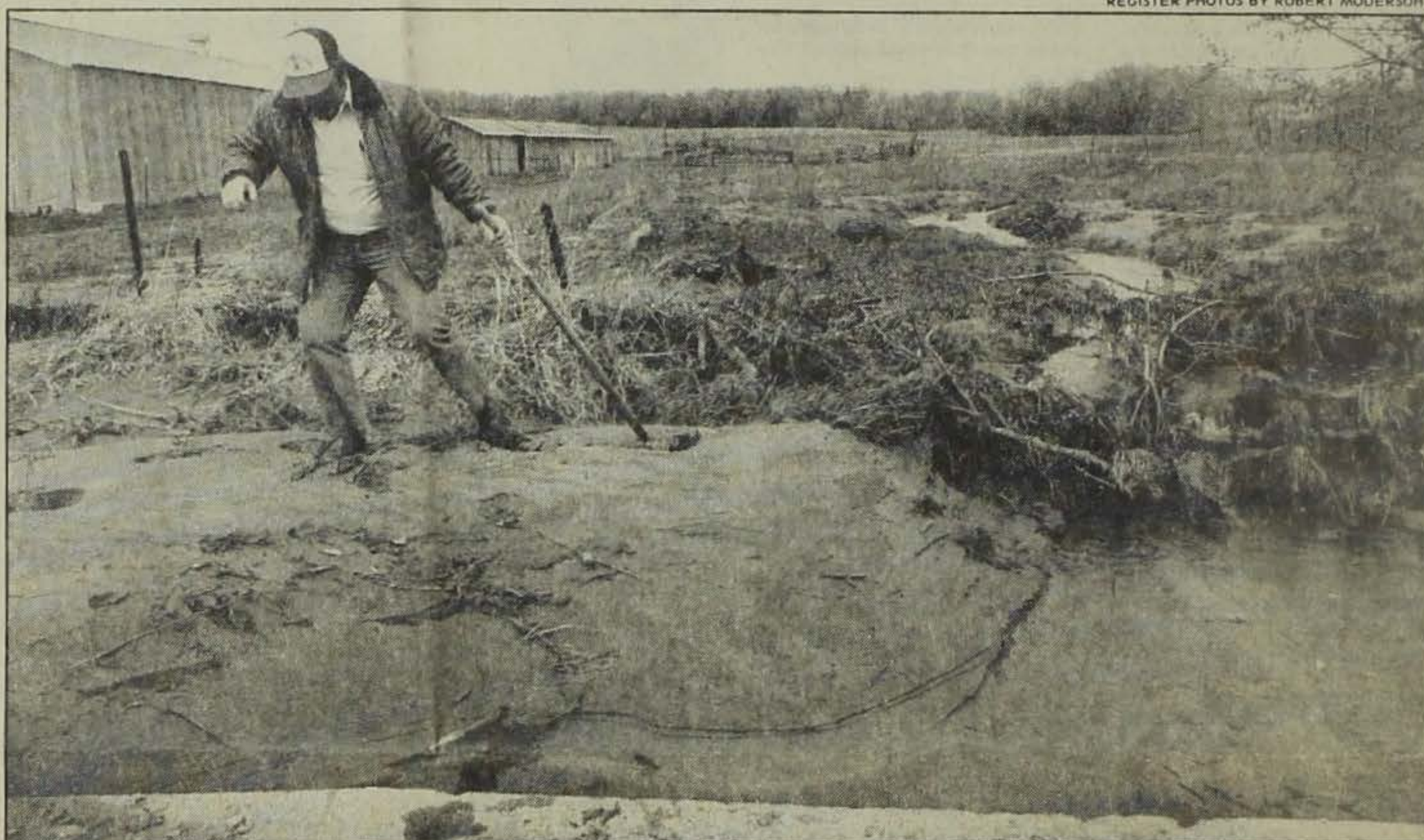
Tama County employee Dwight Surber sinks into silt caused by erosion, which also has led to several accidents near this Chelsea roadside.
