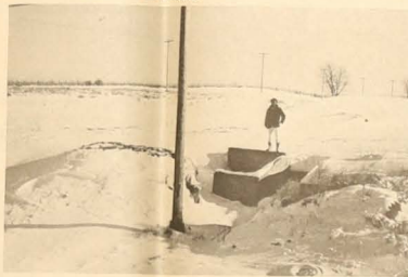
EROSION CONTROL —Conservation Technician Bill Haugh examines a three-foot erosion control drop spillway structure, recently completed on the North Fayette High School property. It was constructed by the industrial arts class of North High. The purpose is to eliminate a gully cutting back across the field.
