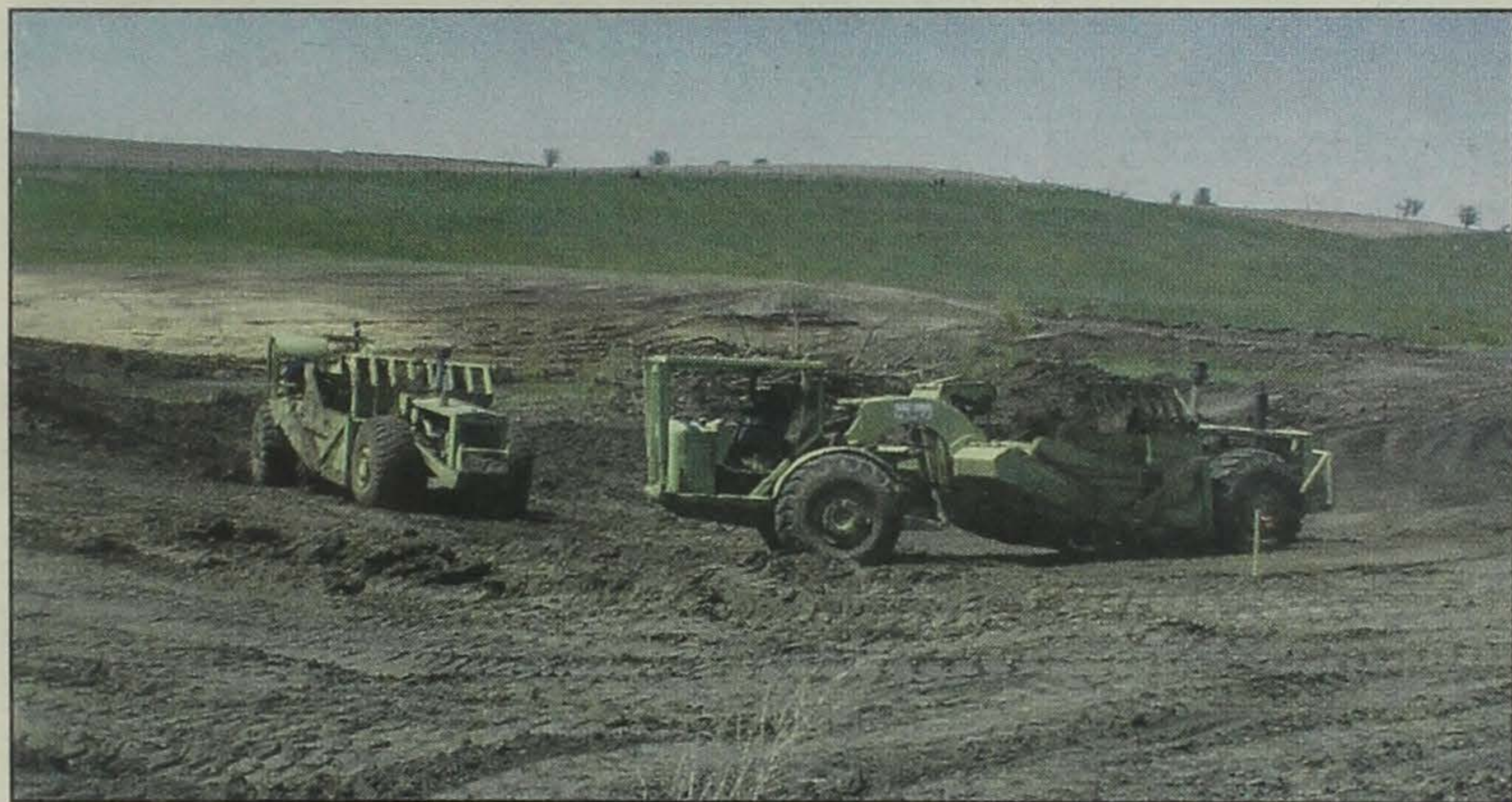
(Above) Construction begins on the grade stabilization structure between the Joe Ballensiefer and Jim and Kathie Mailander farm near Wiota.
