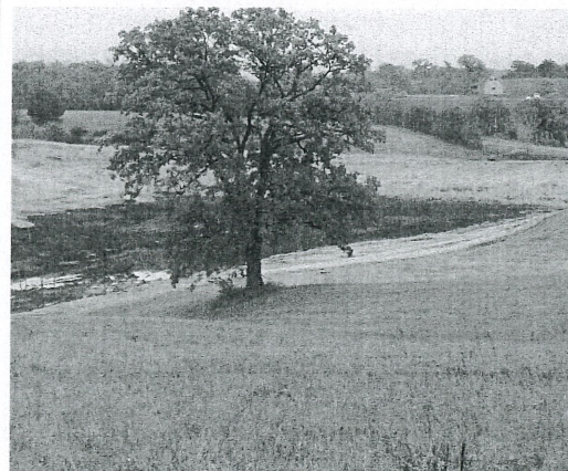
Last year 4 Soap Creek structures were completed like this one located on the Randy Appleton farm. Randy has added some special features to his structure
