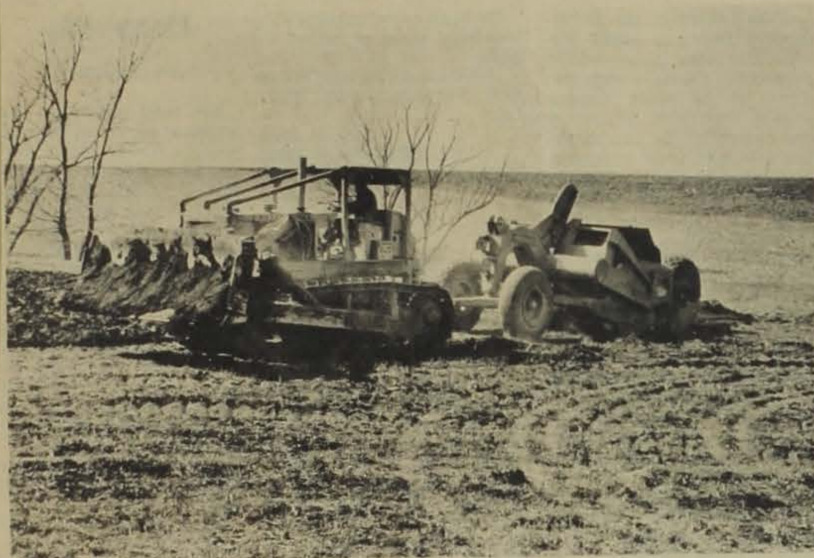
Construction of conservation practices got a good start the last two weeks due to the dry weather. Paul Sanders is shown as he is building a diversion terrace on the Richard Barr farm in Knox Township.
