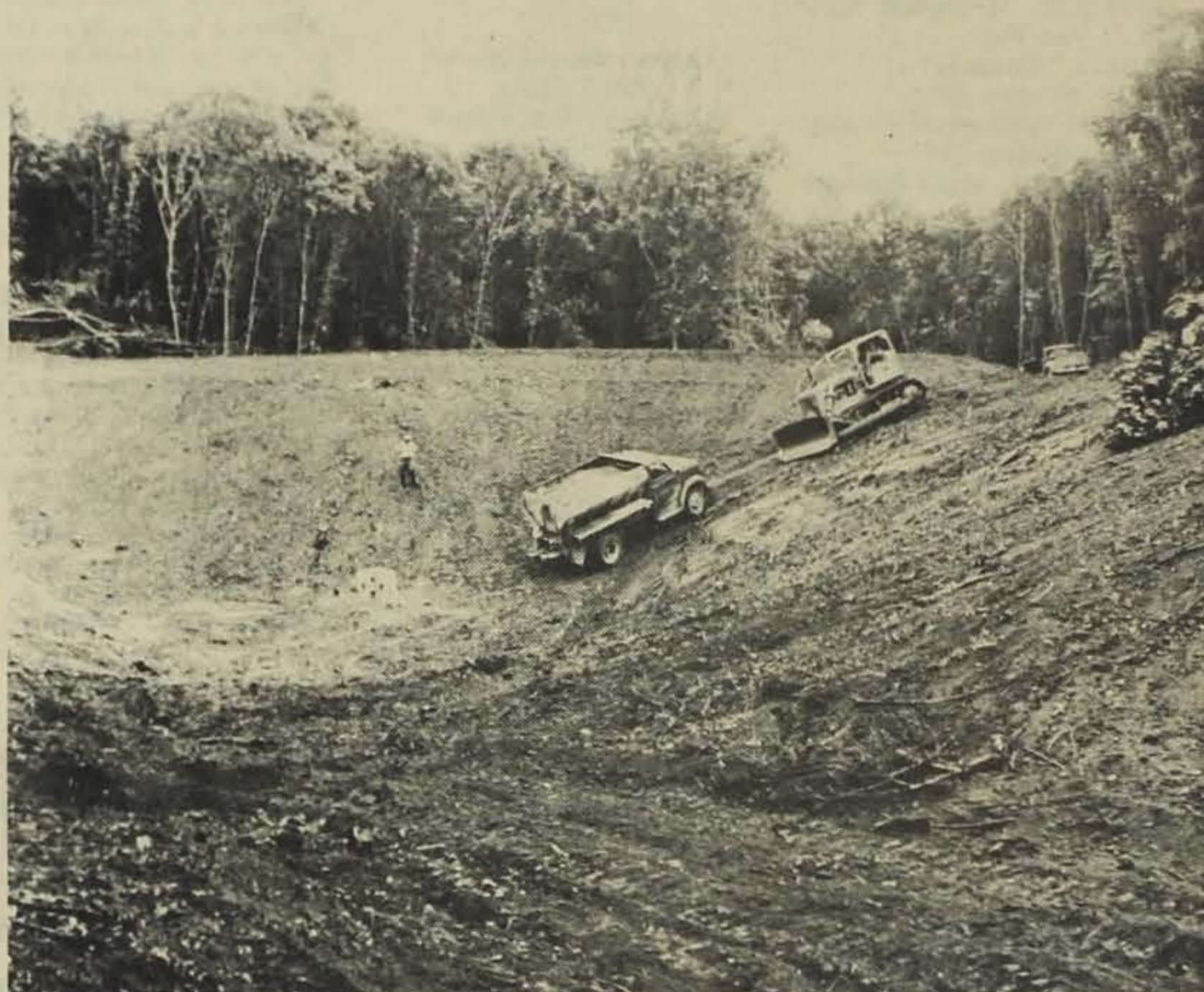
RECREATIONAL FACILITY: Frank Townsend, on the cat, is helping Earl Mateer get a load of rock to the bottom of this new pond for a filter system. T. J. Laing, Soil Conservation Service Technician, is standing on the dam directing traffic.
