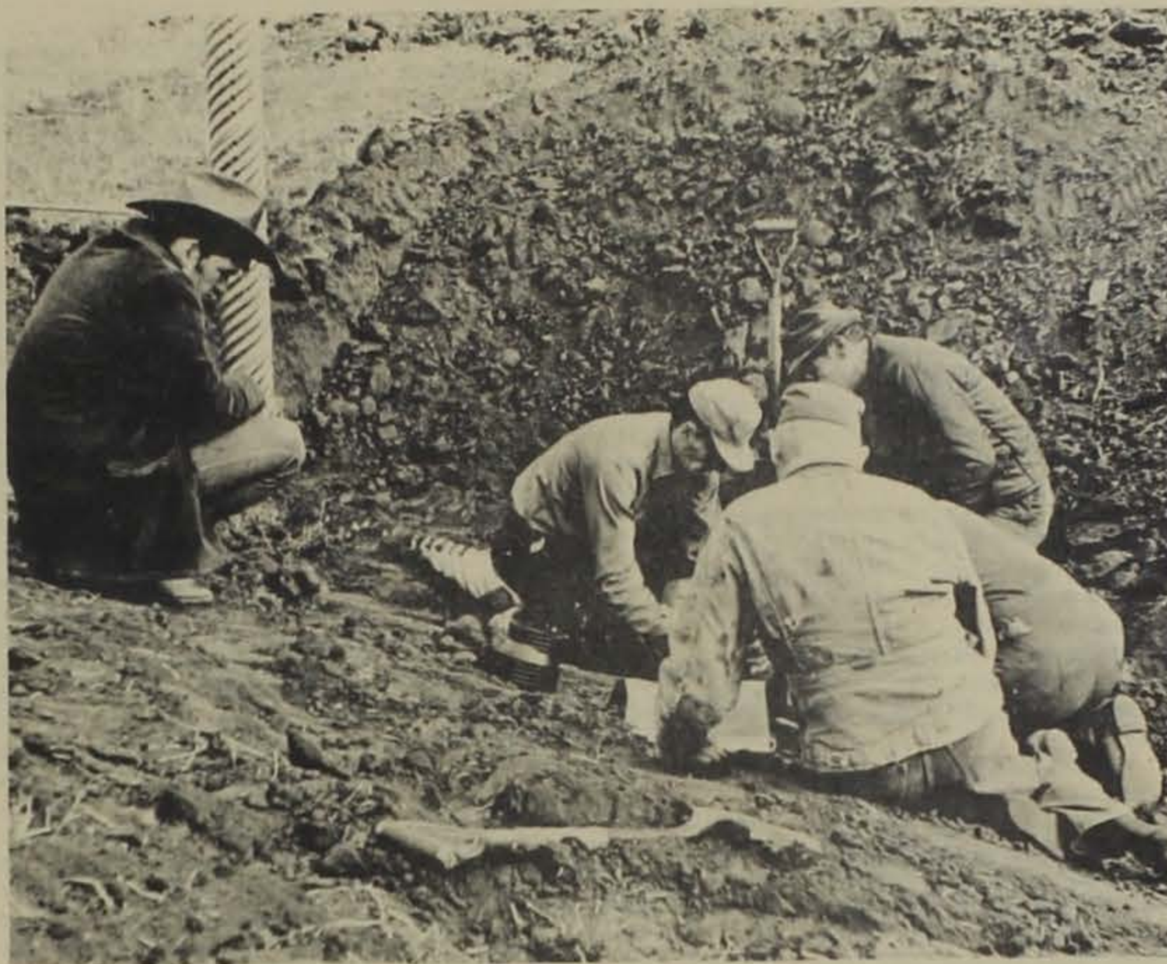
OUTLET DIVERSION: Interest is centered around the activity of installing an intake pipe for a tile outlet diversion on the John Audlehelm farm. Five inch plastic tile is being attached to
