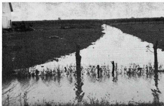
Dwight Glick farm, Maine Watershed. Here is the type of drainage ditch which will remove the water shown above and make these areas more productive. Outlets sometimes require cooperation with a neighbor or County Board of Supervisors.
