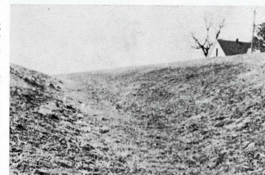
A sod-waterway on state highway property along the highway east of Numa. Steep waterway was seeded and mulched and the bottom area was hand sodded. As you can see, it has held very well.
