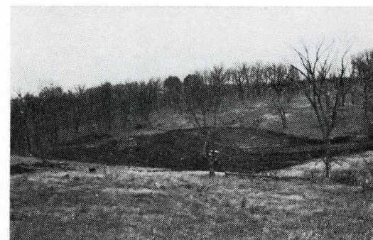
A second structure is being built on the Arthur Jay farm, Moulton Watershed. This structure was located to control gully erosion and to provide a crossing for livestock and machinery.
