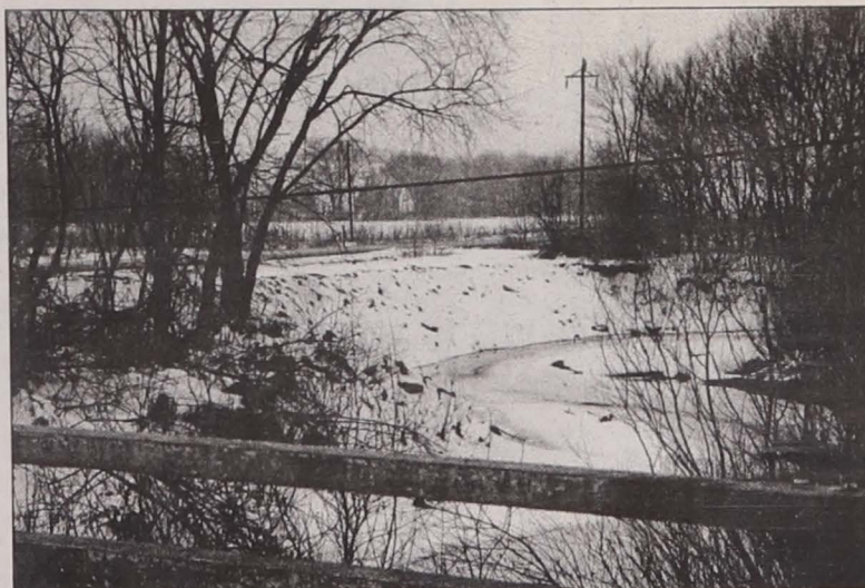
A streambank stabilization project was completed on Robert Yaeger's farm along Flint Creek in Pleasant Grove Township. Riprap was installed to prevent the creek from eroding away the bank. This project will also include riparian buffers, filterstrips and wetland areas. The Des Moines County Soil and Water Conservation District is partially funding this project through a grant received from EPA.
