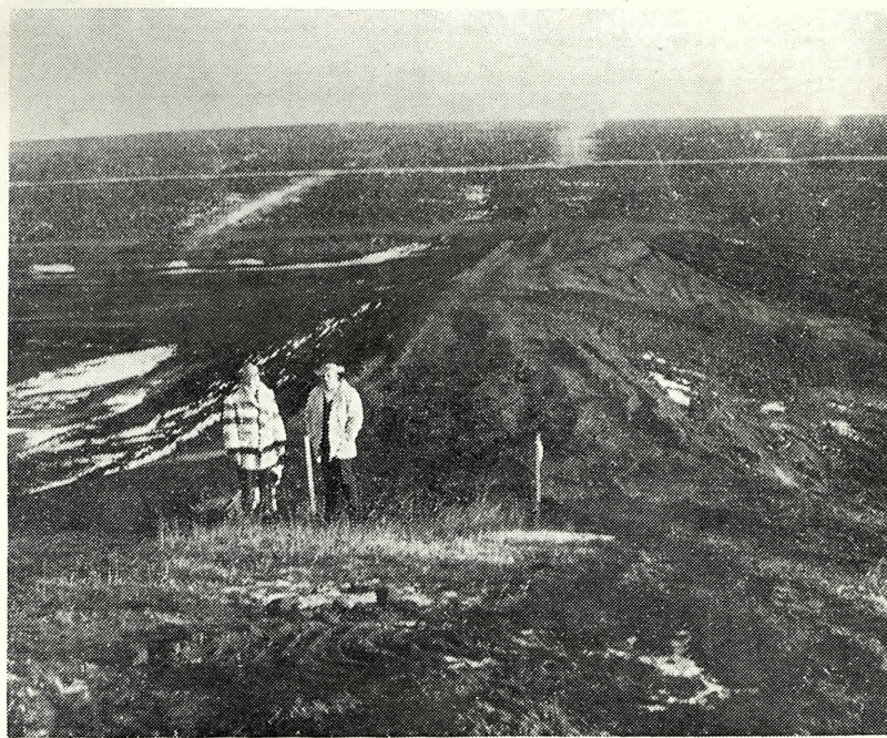
Earl Mickelson and son standing on fill of new dam on the "No View" farm north of Battle Creek, Iowa.
