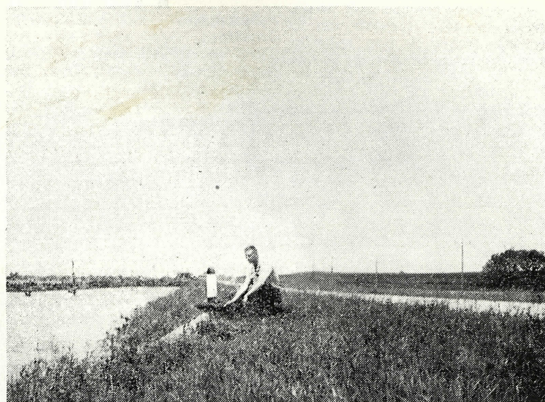
Bruce Marcue inspects flood damage on the Maple River east of Battle Creek.
