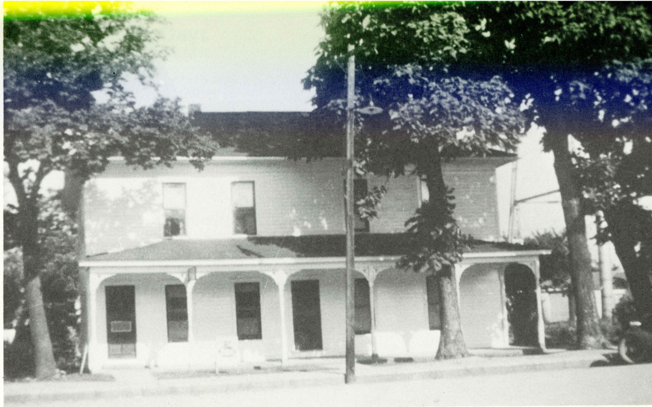
Rhodes Hotel on east side of Main Street, which had many owners, was also, restaurant, apartment house and nursing home.
