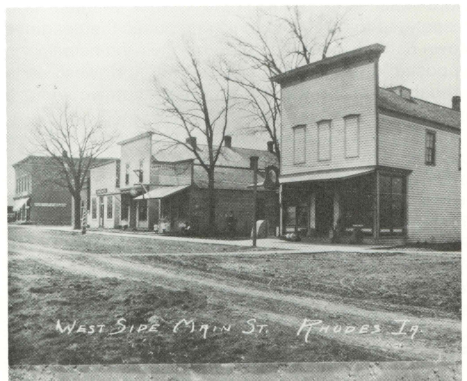
West side, Main Street looking south.
