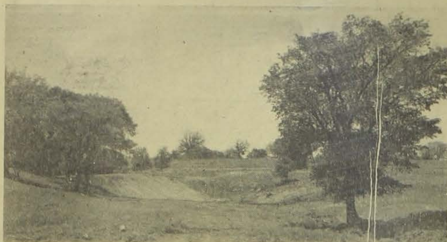
An erosion control structure completed this month on John Spencer's dairy farm just south of Albia will stabilize gullies that were cutting into cropland and toward farm buildings.
