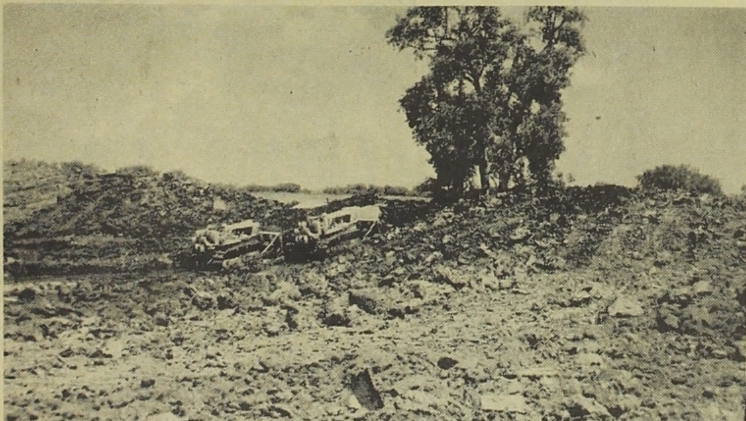
Pictured above are two Ellison caterpillars completing the building of a farm pond for Miss Edna Gray, Bluff Creek township. The building of this pond required the moving of 3900 cubic yards of dirt.
