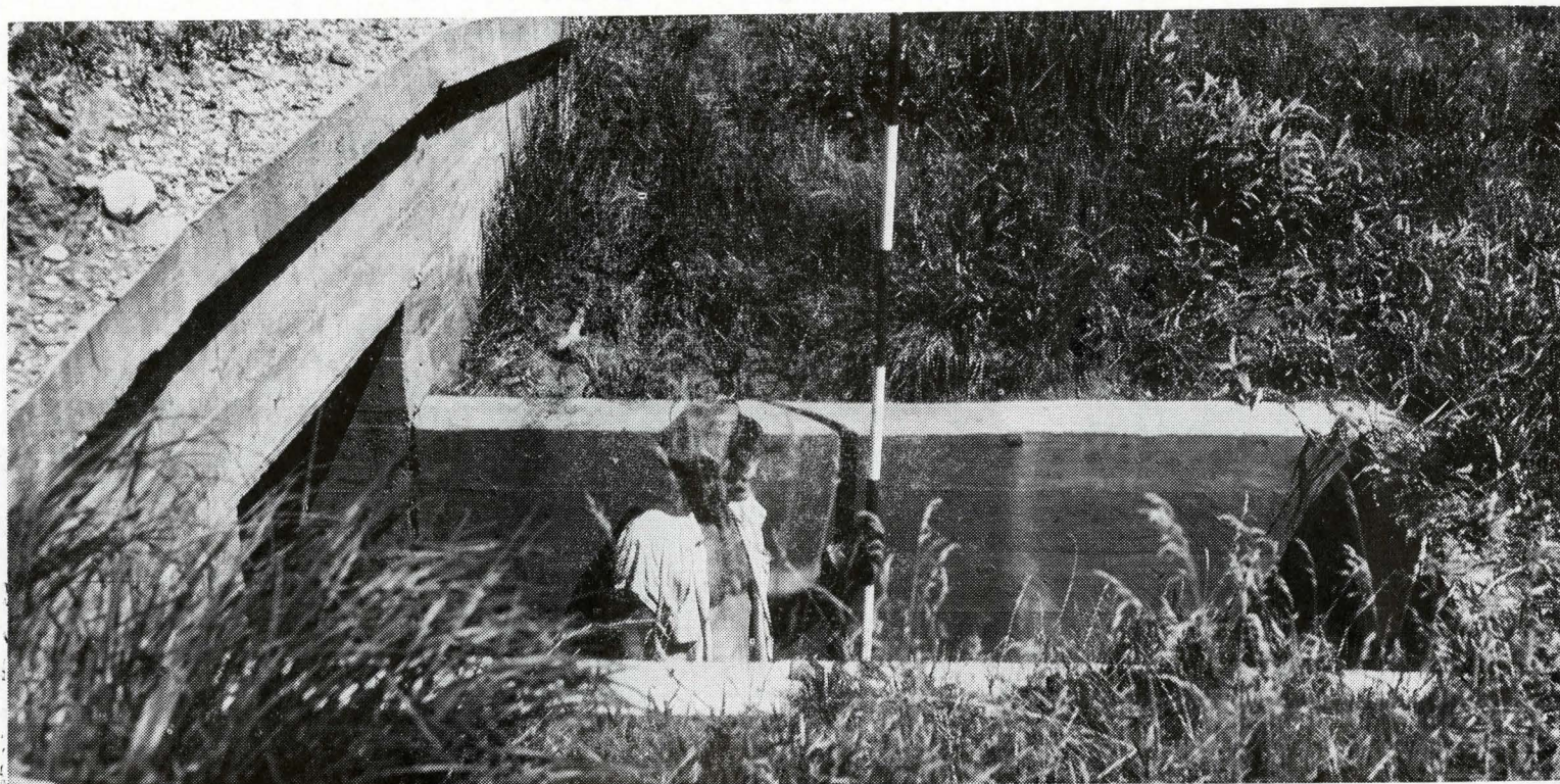
WILBERT LOEB STANDING IN HIS REINFORCED CONCRETE RISER
