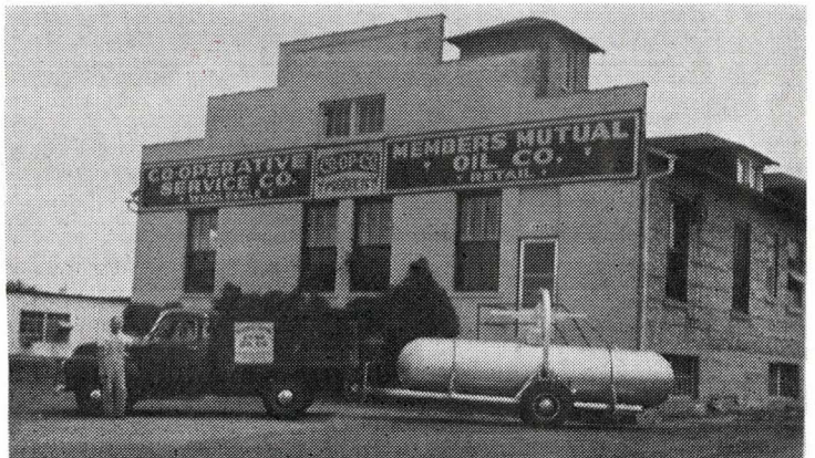
MERL JACOBSEN, Propane Sales and Service
