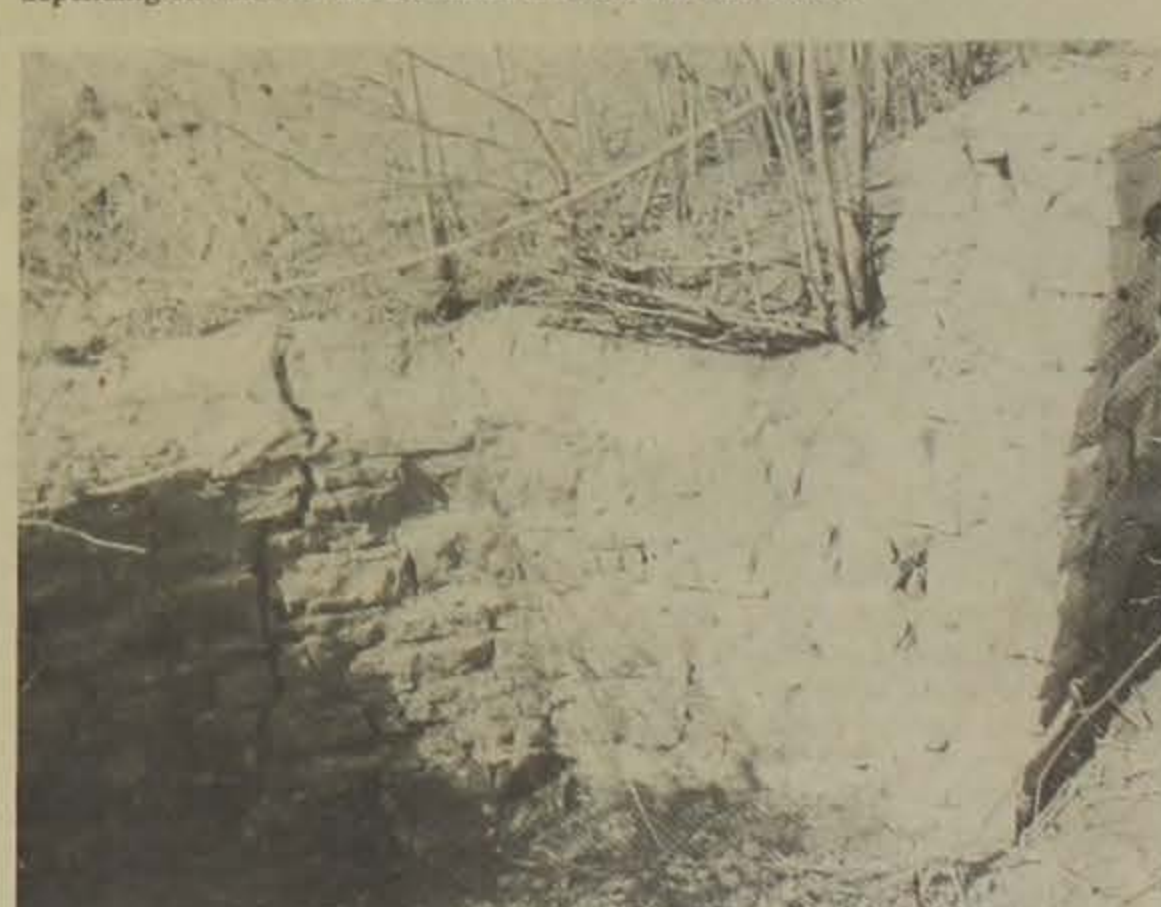
Erosion control practices such as this gully control structure south of Eldora were built by the C.C.C. (Civilian Conservation Corp). The C.C.C. worked in Iowa from 1934-1942. Their work was done by hand with pick and shovel and horses. Even though this structure is approximately 40 years old, it is still in fairly good condition.
