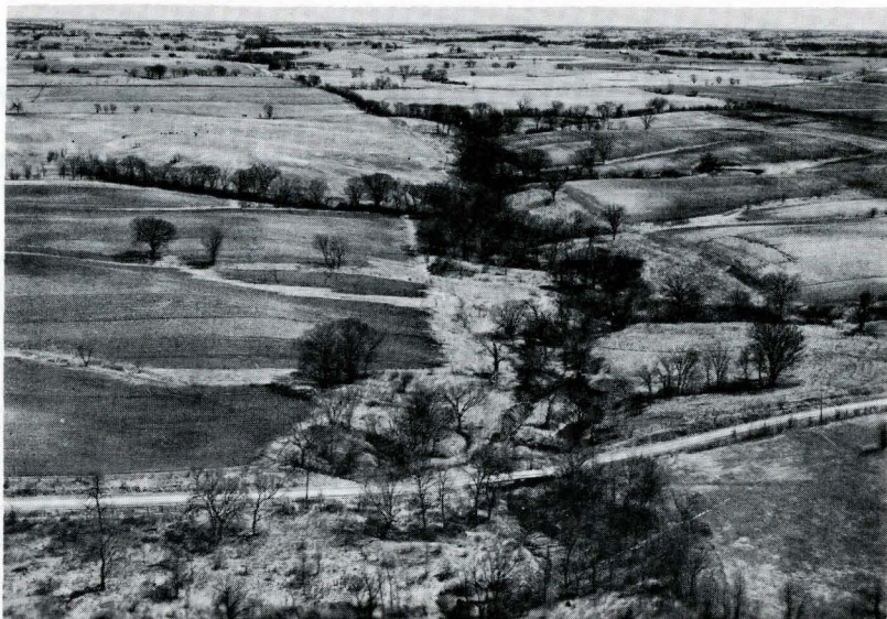
A "Before" picture of E-11 structure site. In June 1964, a hooded inlet, pipe spillway structure was built on the county road in the foreground between the Hubert Morrow and Eugene Houston farms 2 mi. southwest of Moulton. Terraces in the right and background are a part of the land treatment. This is a structure to control the grade of the main waterway upstream from the road. The unsafe, county bridge was replaced by an earth fill and the 18" pipe spillway. (See narrative, top of page 15)
