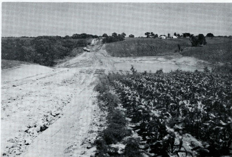
Partial construction picture of the hood-inlet structure on site E-11, Moulton Watershed, looking north along county roadway toward structure site. This is second of this type located on county roads within the Moulton Watershed.
