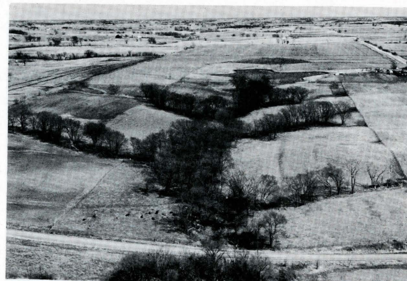
A "Before" picture of D-10 structure, a drop inlet to be built on the county road in the foreground adjacent to the Marvin Stansberry farm 2\frac{1}{2} mi. southwest of Moulton. Pond and terrace in background are part of the land treatment. This structure will control the active gully eroding upstream from the road.
