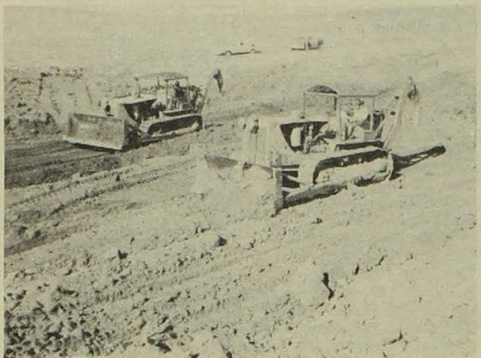
Bulldozers moved the earth in building the dam which was a joint project of Harold Johnson and Richard and Roscoe Woodward on their Cass Township farms.
