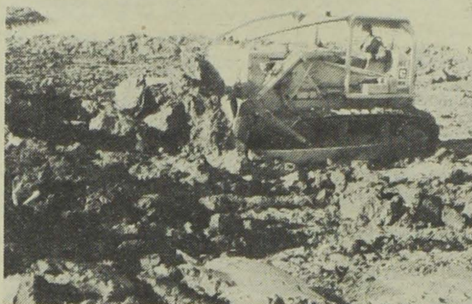
Good topsoil is stockpiled before the terraces are built from subsoil.
