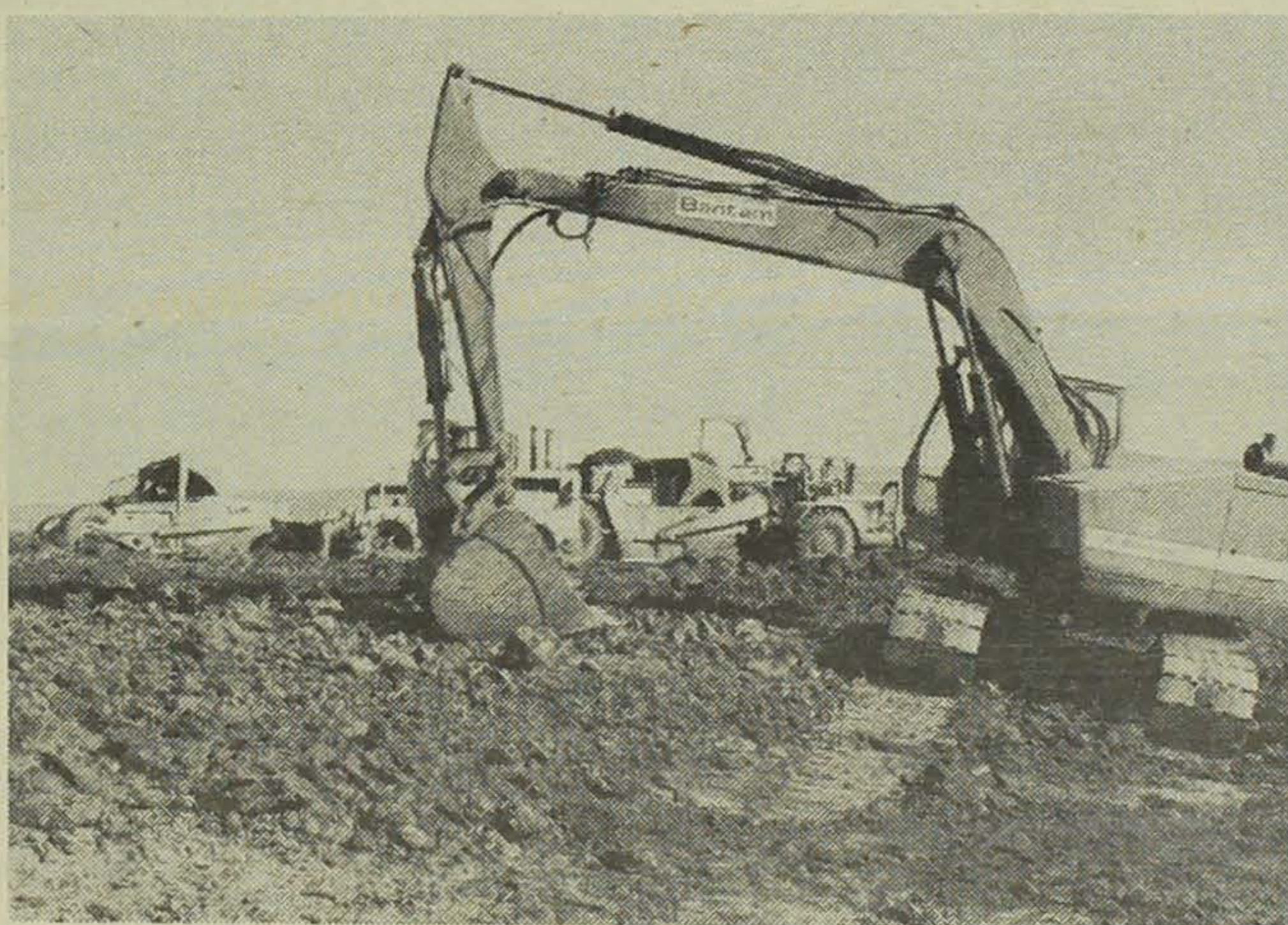
A variety of heavy earth moving equipment is needed to build soil conservation structures. Saxton Inc. of Lenox was given a contract to build seven structures in the Turkey Creek Watershed for $326,773. Some of the equipment is displayed at this work site.
