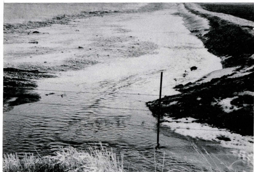
Diversion terrace in operation. Ralph Phillips farm two miles south-east of Montezuma.
