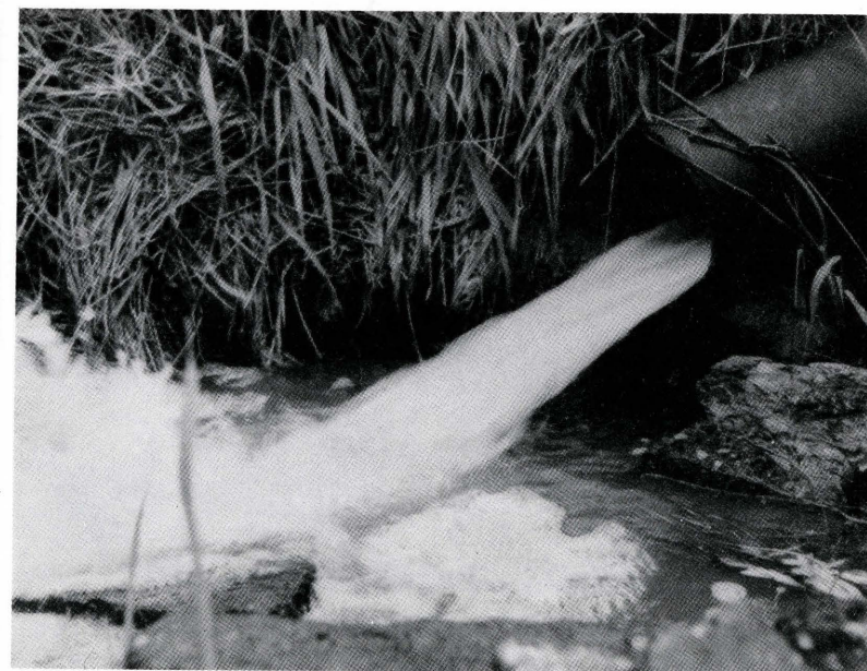
Rains in 1965 really put pond spillway pipes to test. This photo is of the Rex Pitman pond, 5 miles east of Montezuma.
