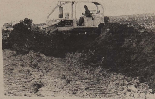
The picture above is an example of a contractor replacing topsoil over a "borrow" area during the final stages of terrace construction. Three types of terraces are generally built in Tama county and include the broadbase, the grass backslope and narrow base.
