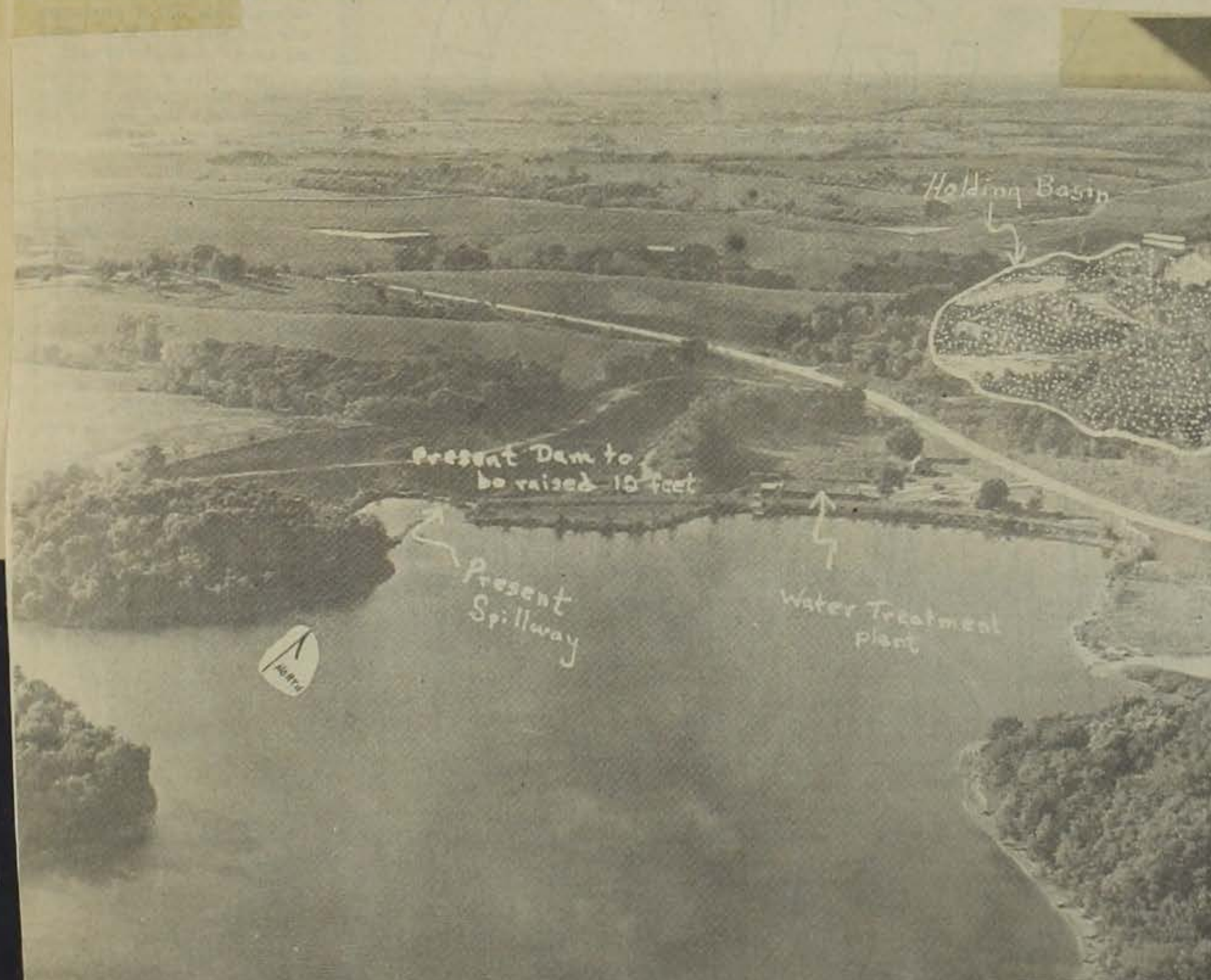
WEST DAM PROJECT: In a photo taken August 11, results of some earthwork are evident prior to raising the dam 12 feet in height. A temporary dam, depicted by two lines, is shown in the upper right hand corner of the photo. The area outlined by dots is the holding basin that will result for water siphoned from the
