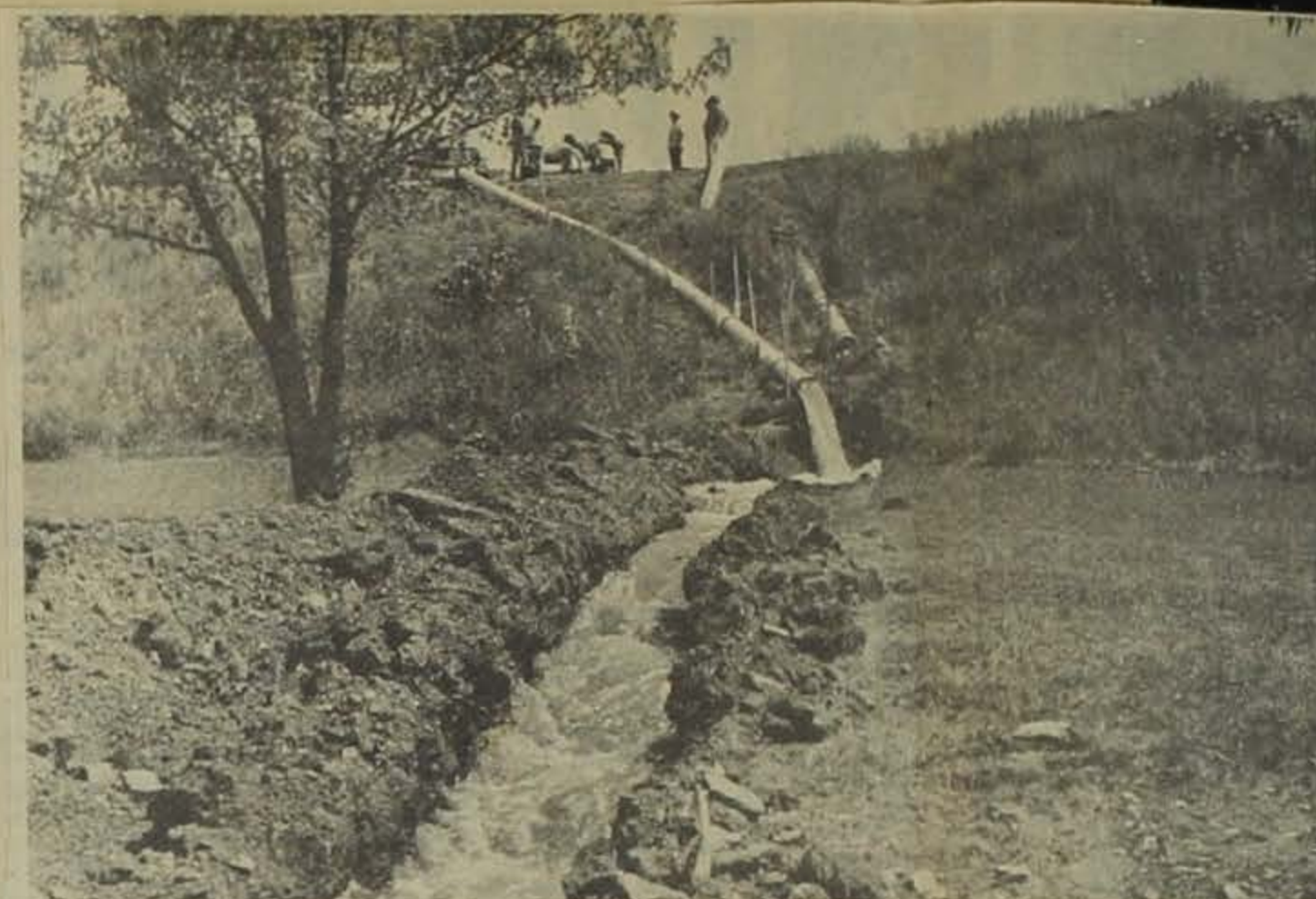
DRAIN LAKE: One of two pipes is shown siphoning water from West Lake Reservoir down to the holding basin below. If all goes as planned, West Lake should be dry by next week and work
