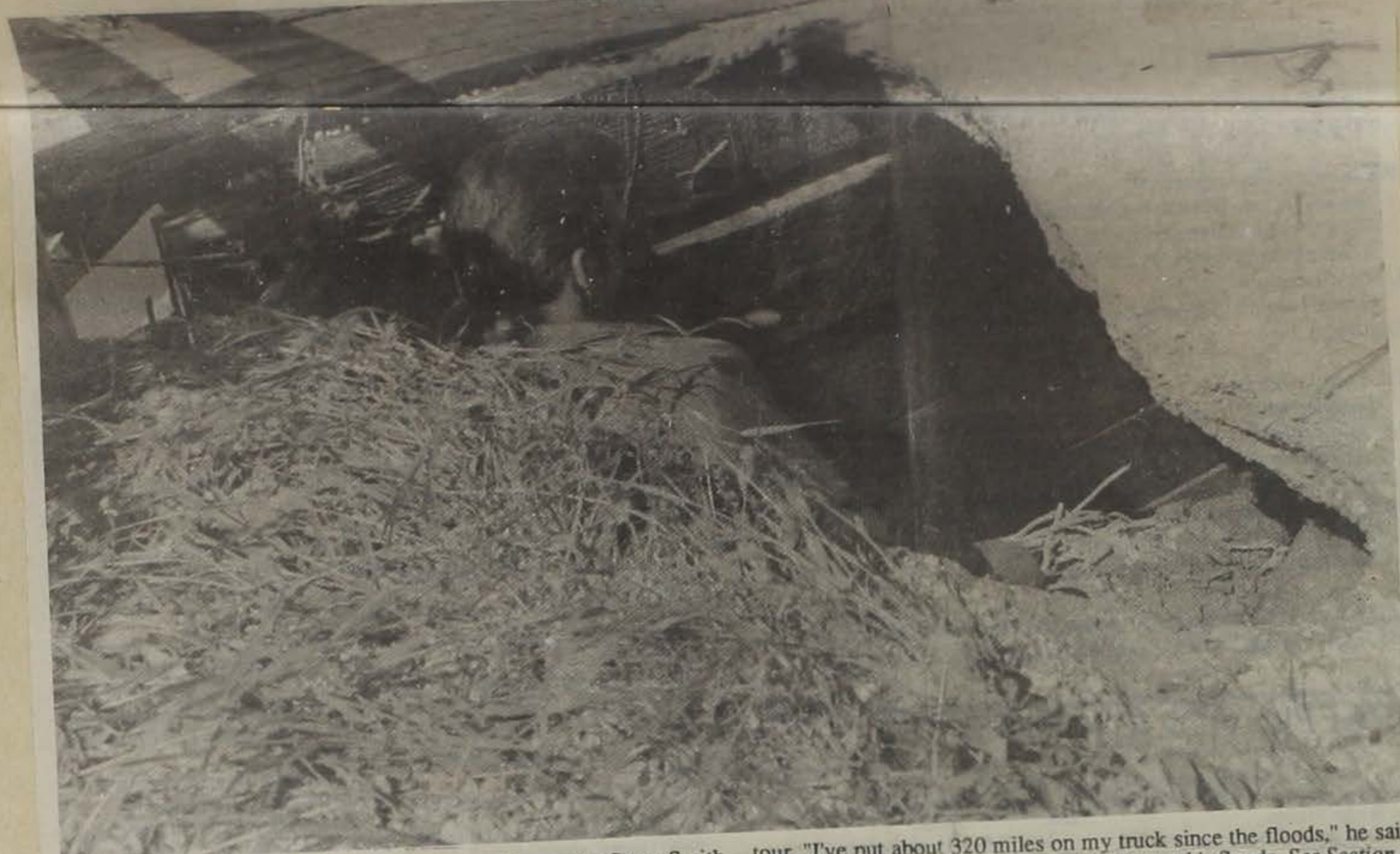
IN OVER HIS HEAD: Clarke County Supervisor Steve Smith inspects a washed-out bridge during another flood damage assessment
