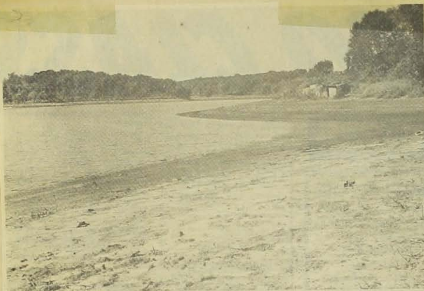
SHORELINE: The receding waters in West Lake give the appearance of a beach—almost. Siphoning of the water in the West Lake reservoir proceeded last week in preparation for making the dam higher. As the water level
