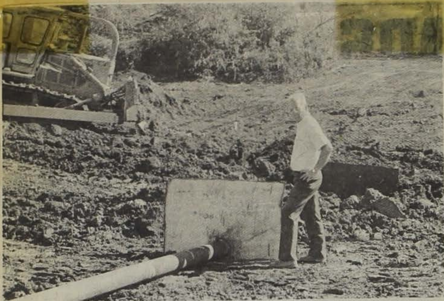
EROSION CONTROL: Lloyd Querrey, owner of land in Section 21 of Ward Township, 2 1/2 miles west of Osceola, looks over the erosion control dam project under way on his property. Andrew Brothers installed a principle spillway
