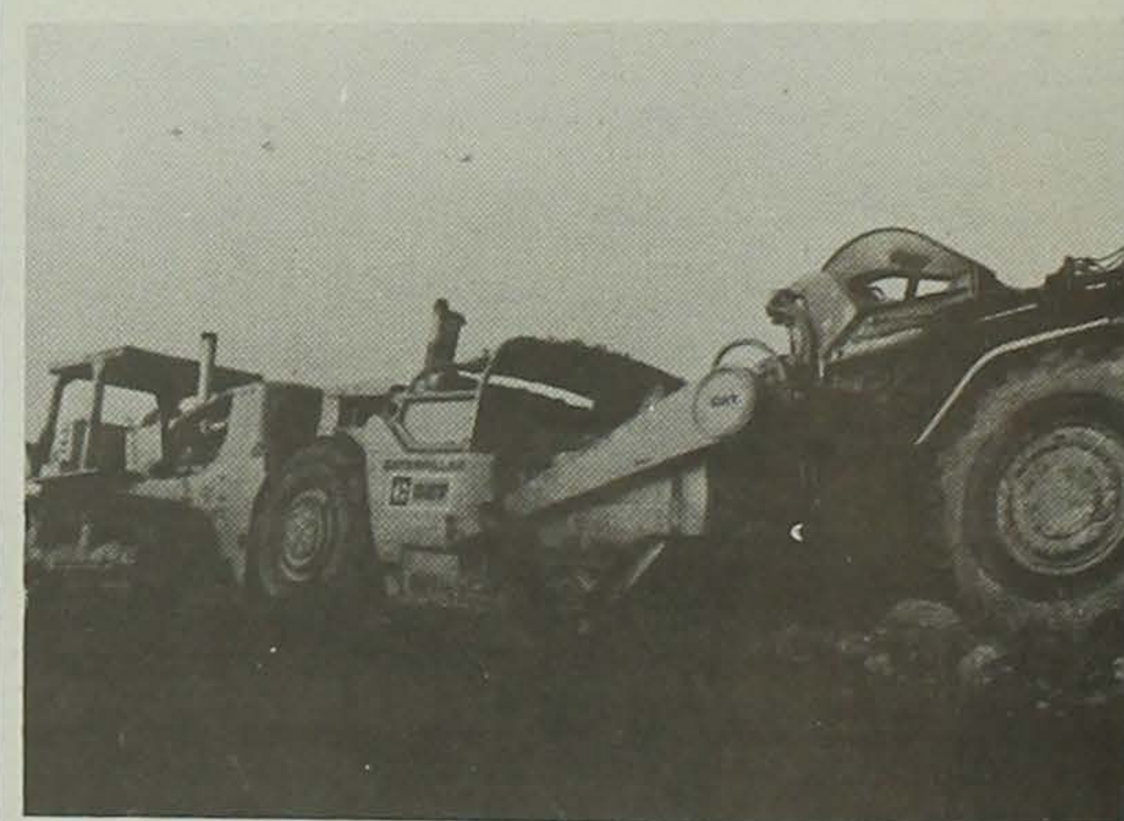
More than 160,000 cubic yards of dirt will be moved to build the six new ponds in the Turkey Creek Watershed. More than half of the needed dams have now been built to control gully formation and downstream flooding.
