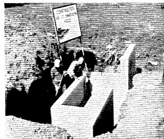
Type A erosion control structure built on the Wm. Kaderavek farm in Honey Creek township. Ronald Ahrens, contractor from Harper, is tak- ing off the last of the forms.
