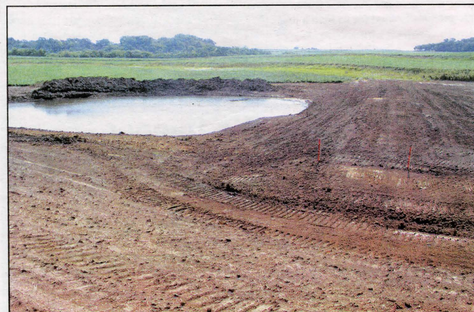
A grade stabilization structure or pond was constructed on the Mark Nelson property, northeast of Clermont. The Nelsons constructed terraces prior to the pond which will reduce sedimentation within the pond, extending the ponds effective life. EQIP, a cost share incentive program, was used to help defray the cost.
