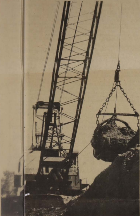
Digging the first cut
