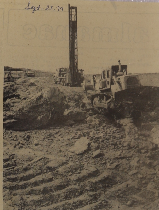
An overburden drill and earth moving machine are operating near the dragline. More pictures on Page 7
