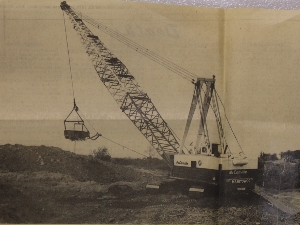
One of the large draglines in operation near Bussey.
