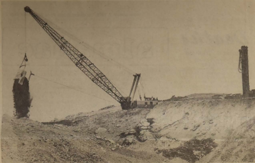
Dragline in operation
