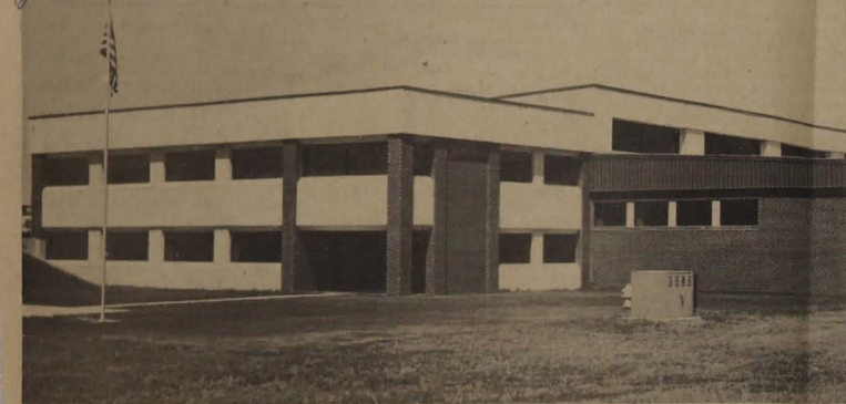
Water treatment plant at Rathbun.
