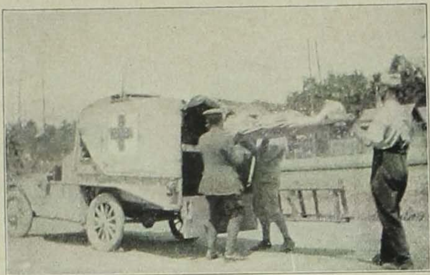
PUTTING IN UPPER STRETCHER
