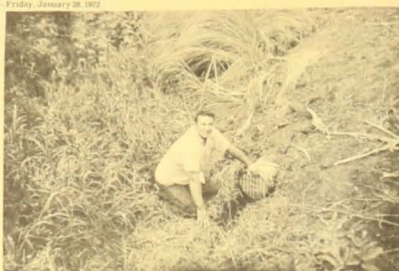
AUGUST PAGEL examines the outlet pipe for a muted system in Fremont township. Pagel and three of his neighbors cooperated to install the life main.
