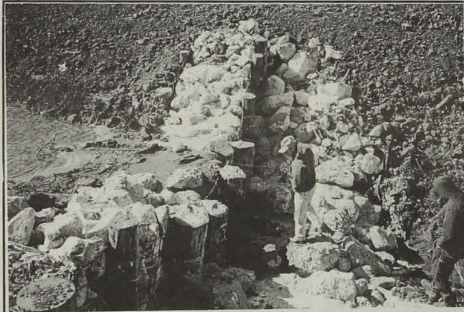
Ron Petesen of the Natural Resources Conservation Service examines a Hungry Canyons structure he designed on the Ed Reinig farm in Shelby County. The structure was made of cattle panels, telephone poles, cable and rock.
