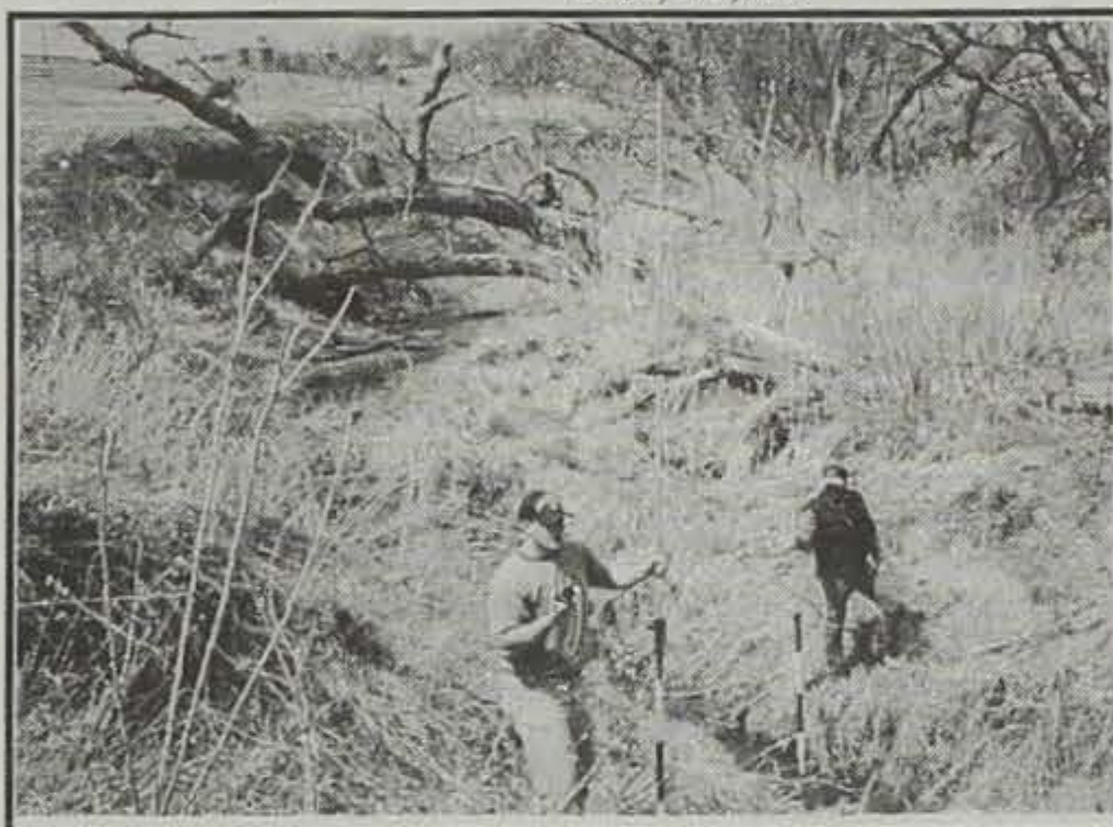
Jordan Lanini and Scott Chapman of the Crawford County NRCS survey a site for a dam in the East Boyer Watershed.
