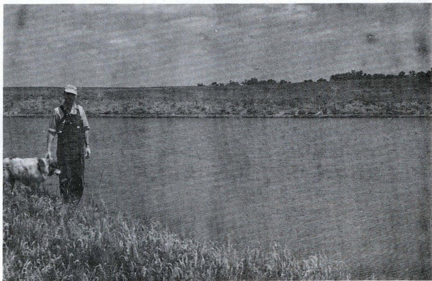
Pond after construction - Ross Mintle farm.
