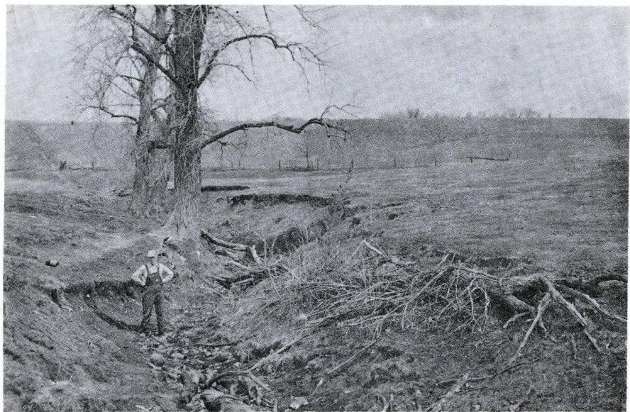
Pond site before construction - Ross Mintle, 3 miles northeast of Grinnell.
