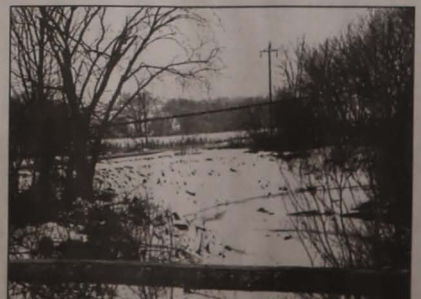
A stream bank stabilization project was completed on Robert Yanger's farm along Flint Creek in Pleasant Grove Township. Rip rap was installed to prevent the creek from eroding away the bank. This project will also include riparian buffers, filterstrips and wetland areas. The Des Moines County Soil and Water Conservation District is partially funding this project through a grant received from EPA.
