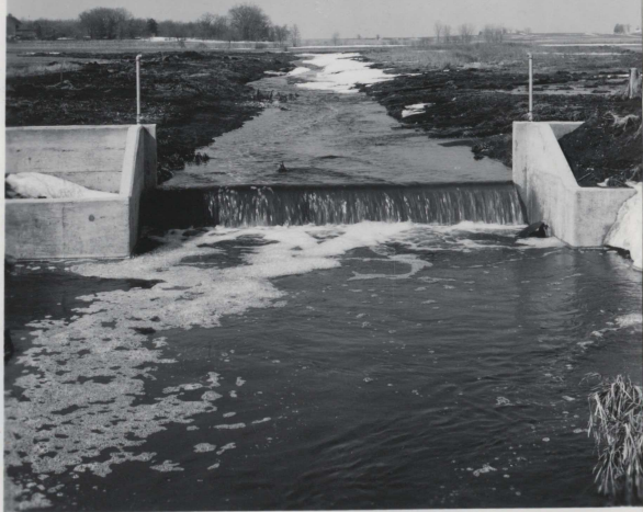
Hoffman/Broghammer concrete structure built Sept. 1959 picture taken 3/31/60
