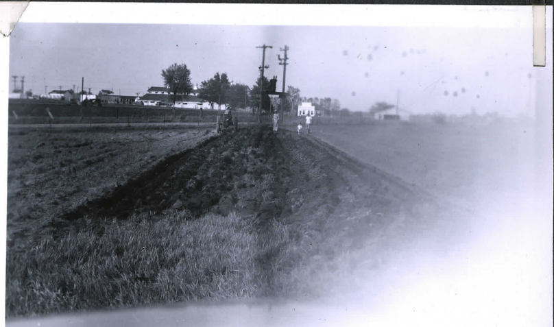
Bickert Farm 5-24-50 Terrace construction with ordinary Farm Plow. Bickert's man on tractor John Botts Bob Judge Ricky Botts
