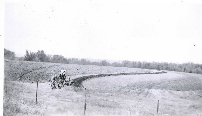
D. Patton Farm Terrace in Field 13 fallon on tractor Referring to add height to terrace
