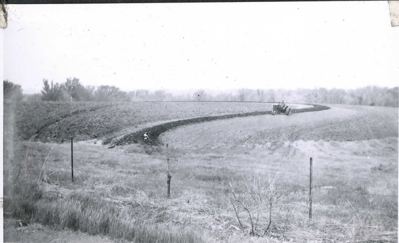
D. Patton 5-20-50 Terraces in field 13 Replowing to add height to terrace.
