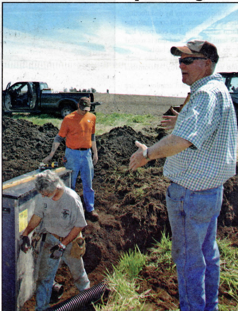
Black Hawk County farmer, Nick Meier, right, watches as technicians install a saturated buffer on his farm near La Porte City. The saturated buffer is designed to remove nitrates and other nutrients from tile drainage water.
