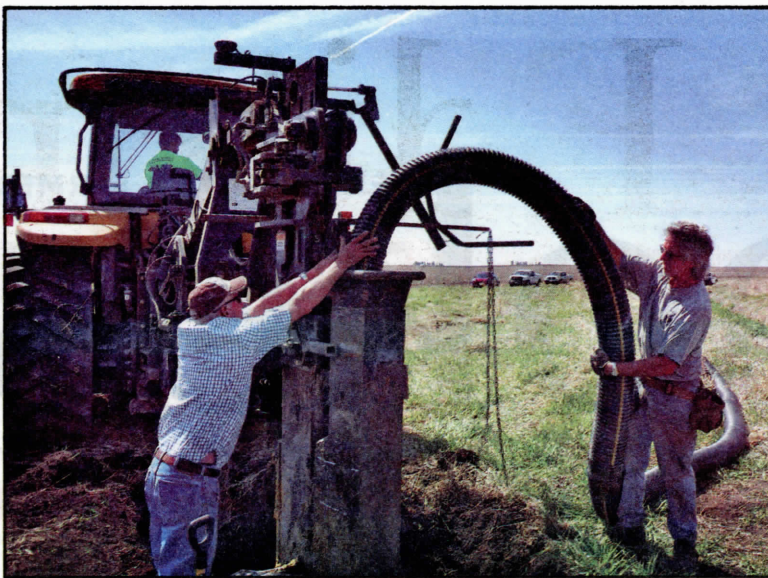
Farmer Nick Meier, left, and Gene Etringer feed a machine installing perforated tile along a buffer strip on Meier's Black Hawk County Farm. The perforated tile is part of a saturated buffer designed to reduce nitrates and other nutrients from tile drainage. PHOTO/DIRCK STEIMEL
